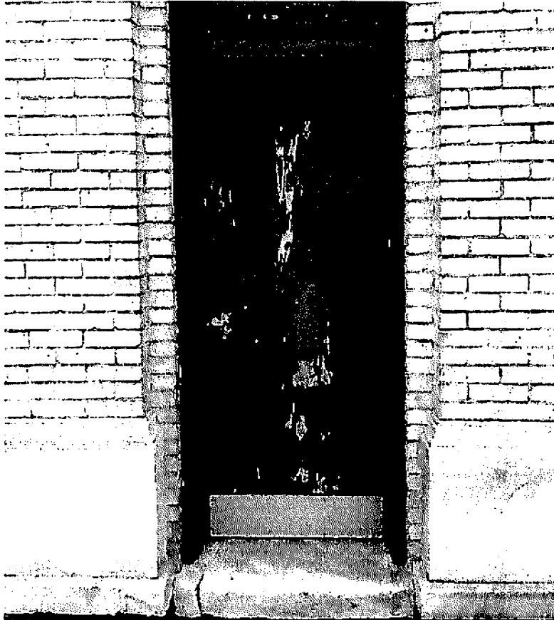
Figure 23: Deteriorating wood door.
