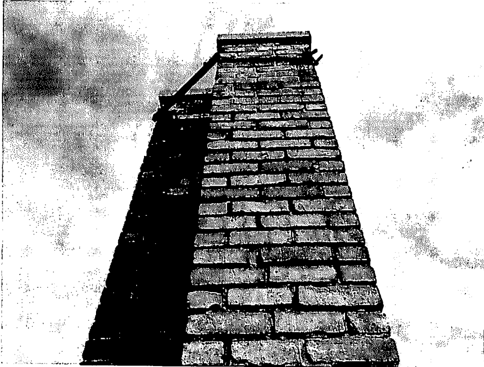
Figure 25: Deteriorated brick at chimney.
