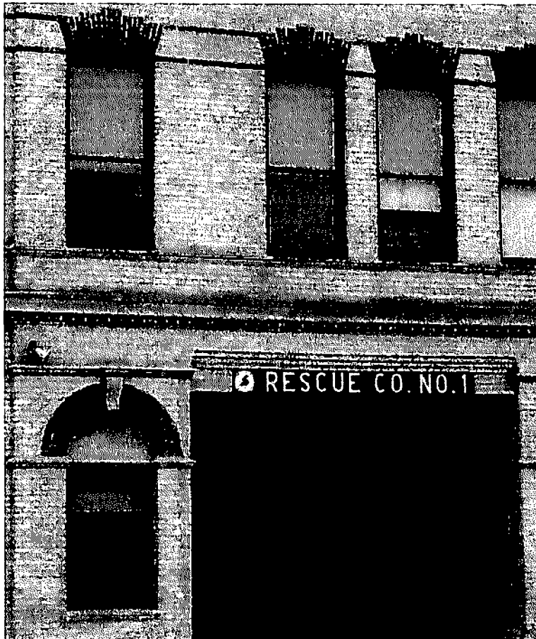
Figure 20: Typical window systems.
