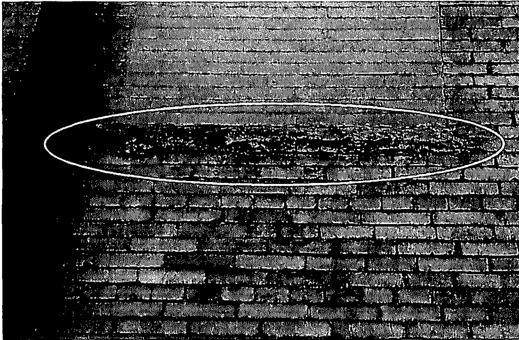
Figure 35: Deteriorated sill.
