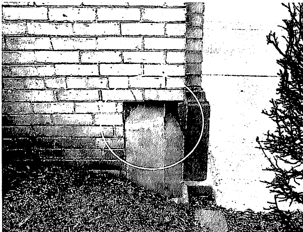
Figure 34: Stone spalling.
