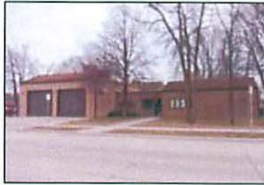
Station 2: 2413 South 18 th Street Rescue 2/Med 2 Trench Rescue Trailer
