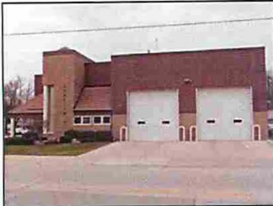
Station 4: 2622 North 15 th Street Ladder 4 Engine 6 (Reserve Engine)
