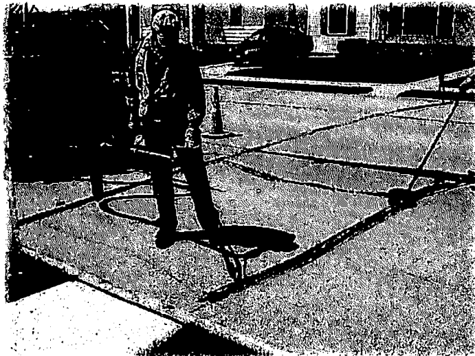
Crack Filling on Asphalt Overlay
