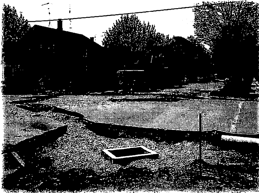
Storm Drain (Catch Basin) Installation
