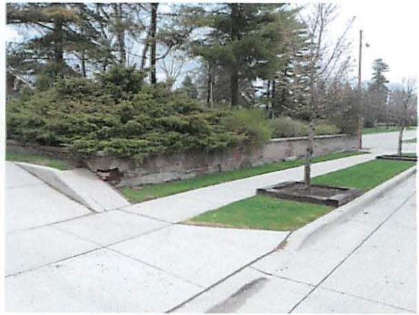
Current Condition Looking NE
