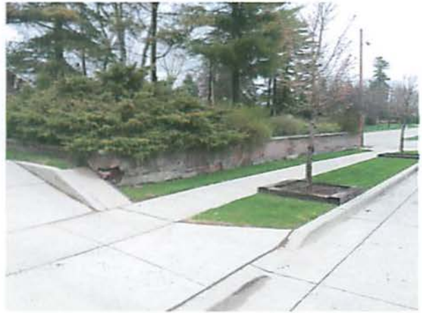
Current Condition Looking NE
