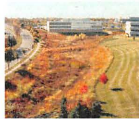
Green Infrastructure bioswale
