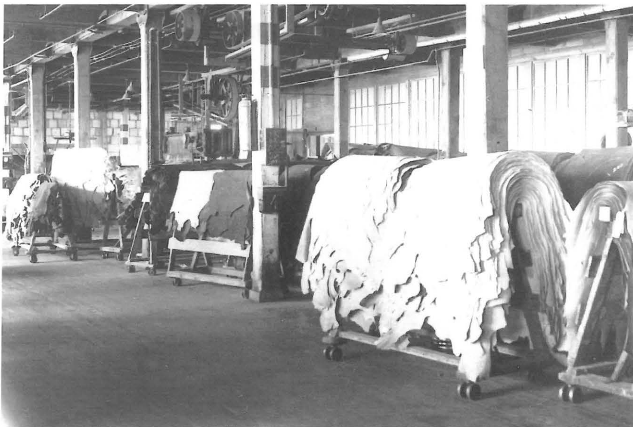
Figure 7: Interior of main tanning sections (Sections 7 and 8), 1932
