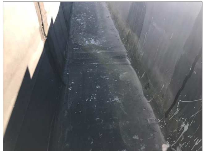
Roof #6 – Overview Photo
