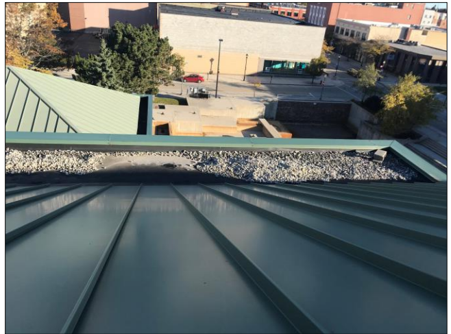
Roof #7 – Overview Photo
