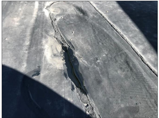
Roof #4 – Area was sealed with polyurethane sealant.
