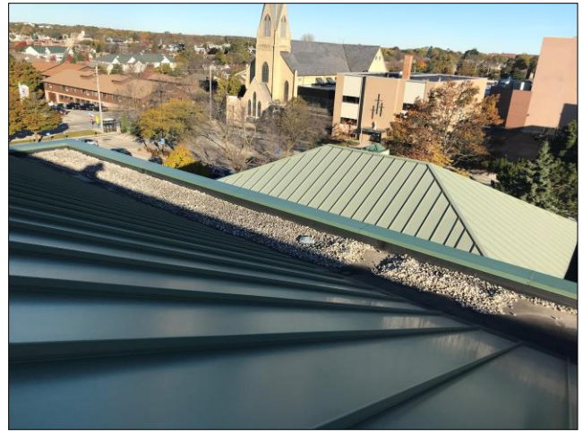
Roof #3 – Overview Photo
