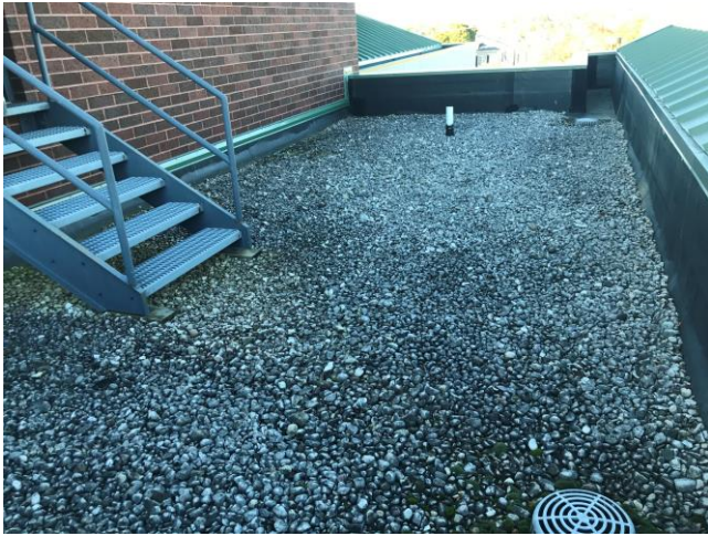
Roof #2 – Overview Photo
