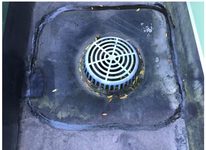
Roof #4 – Sealant applied to delaminated perimeter of target patch.
