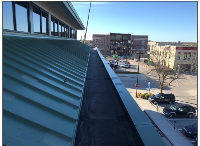
Roof #4 – Overview Photo
