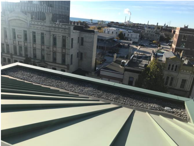
Roof #5 – Overview Photo
