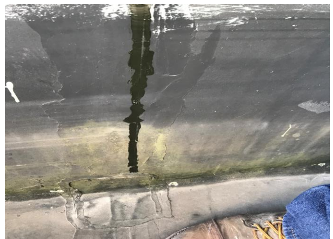
Roof #6 – Cracked lap sealant replaced with new polyurethane.
