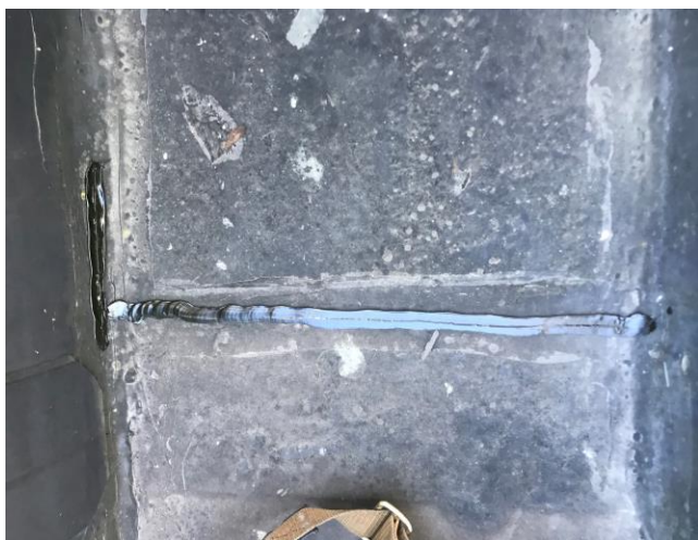
Roof #6 – Sealant applied to cracked and delaminated areas.
