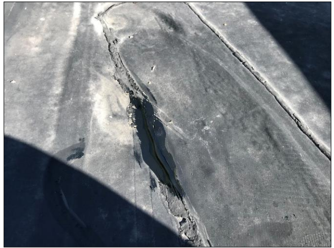
Roof #4 – Area was sealed with polyurethane sealant.
