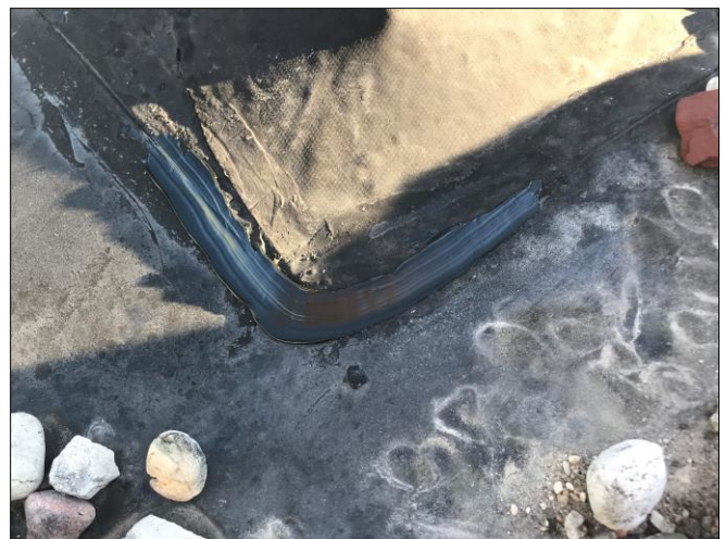
Roof #1 – Area repaired with polyurethane sealant and set back in place.
