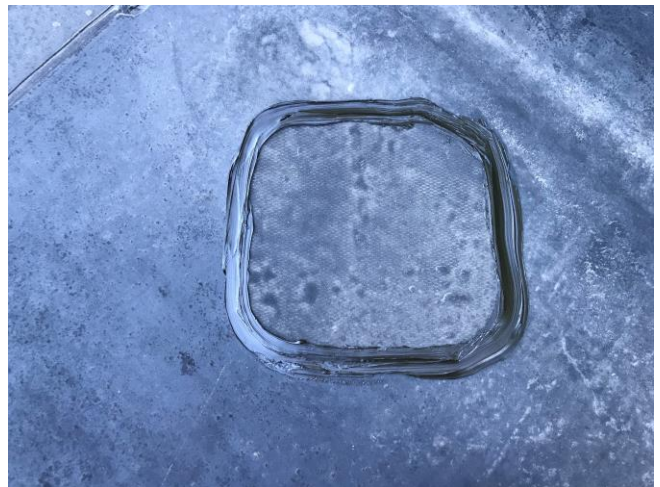
Roof #6 – Sealant applied to perimeter.
