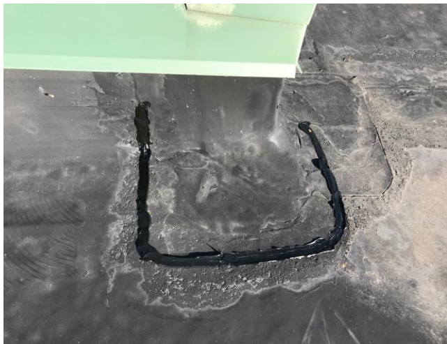
Roof #6 – Sealant applied to delaminated areas of corner flashing.
