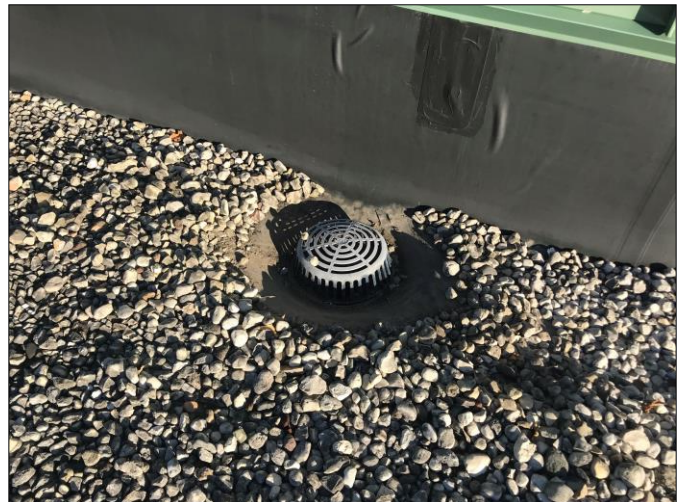
Roof #1 – All drain areas were cleared of ballast and debris.
