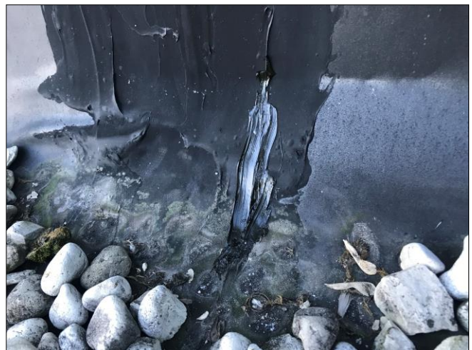
Roofs #1 – Void was filled and sealed with polyurethane sealant.
