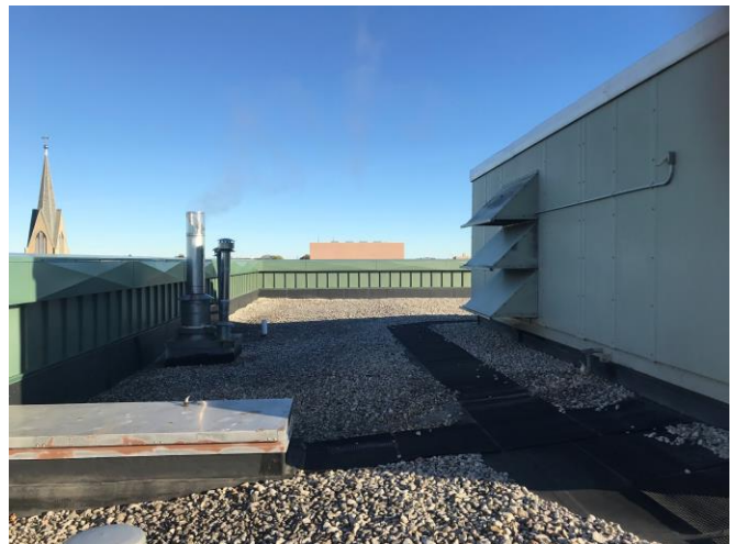
Roof #1 – Overview Photo
