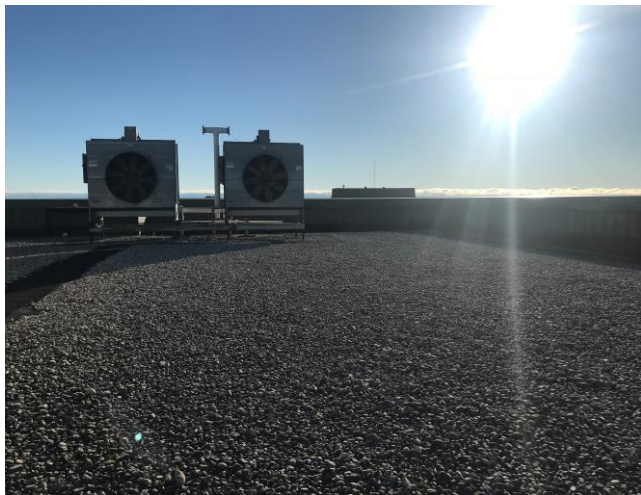
Roof #1 – Overview Photo
