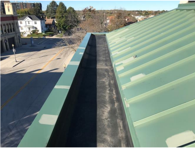
Roof #7 – Overview Photo
