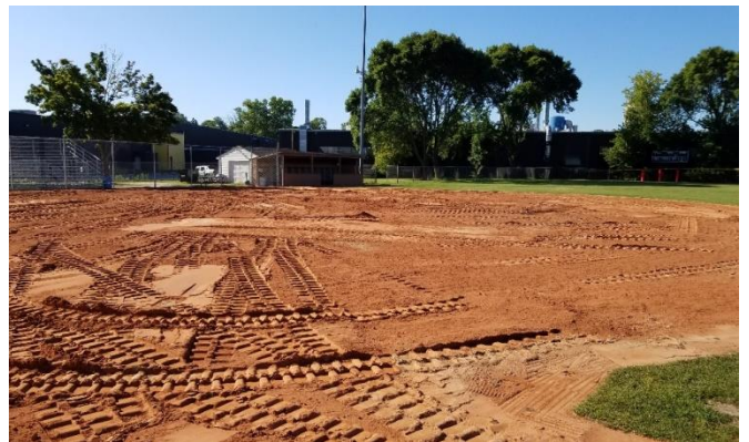
Field Improvements at the Wildwood Softball Complex
