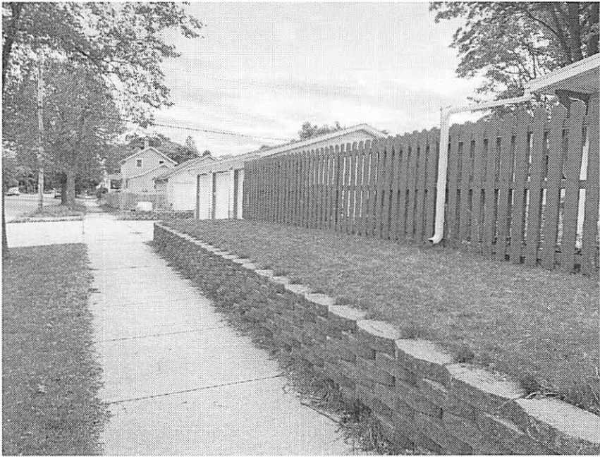
Move fence out to 1' from property line, while maintaining a 10'x10' right triangle from garage end to support line of site from garage AND alley exit.
