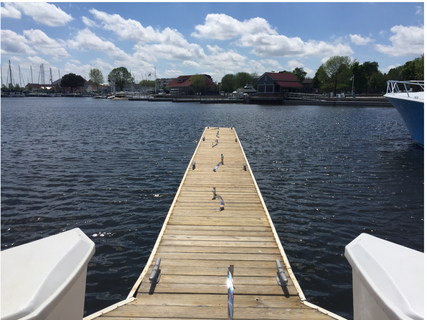
Cleaned G Dock Slip with Bird Tape
