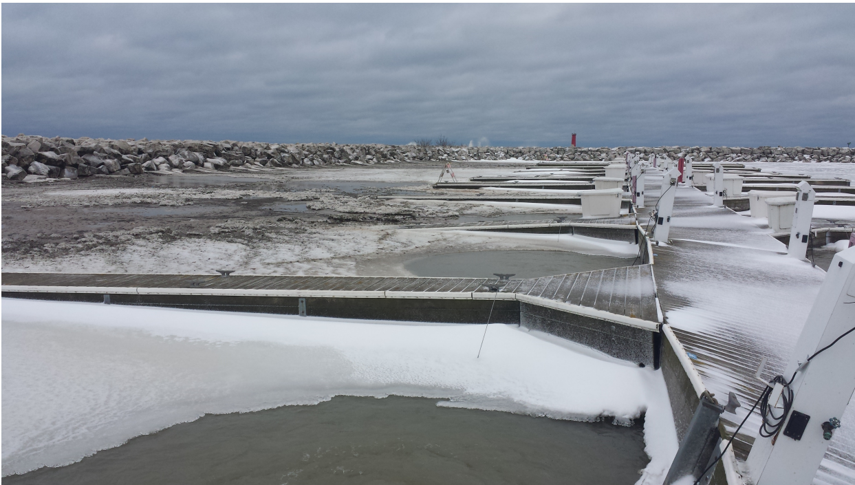
North Break Water looking East from A35
