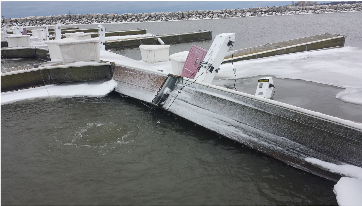
C51 Looking East Southeast
