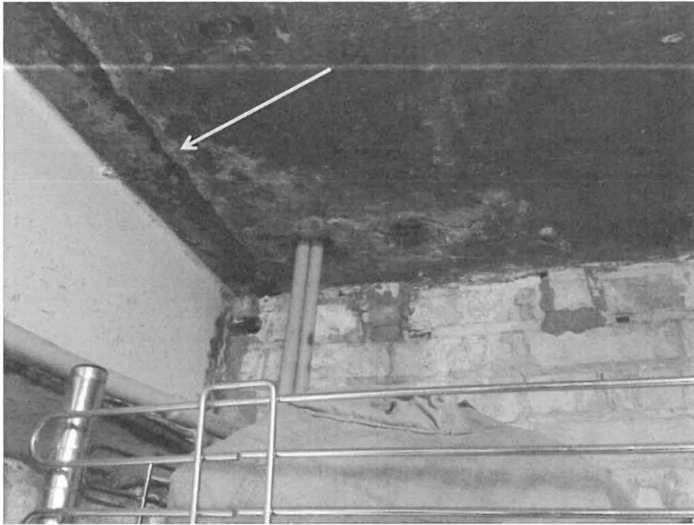
Figure 39: Steel Corrosion.
