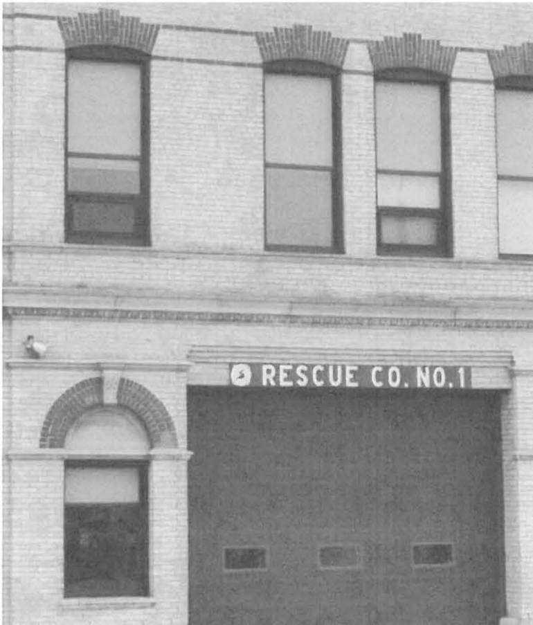
Figure 20: Typical window systems.
