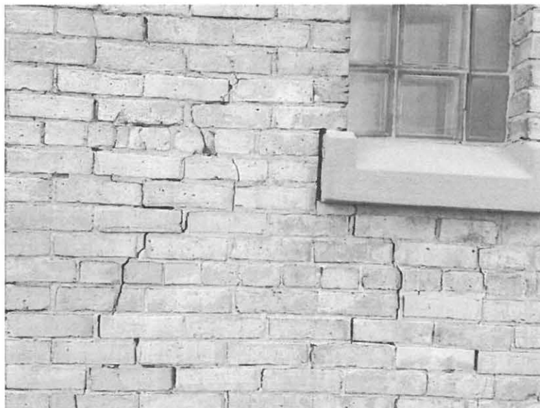
Figure 24: Brick/mortar cracking.
