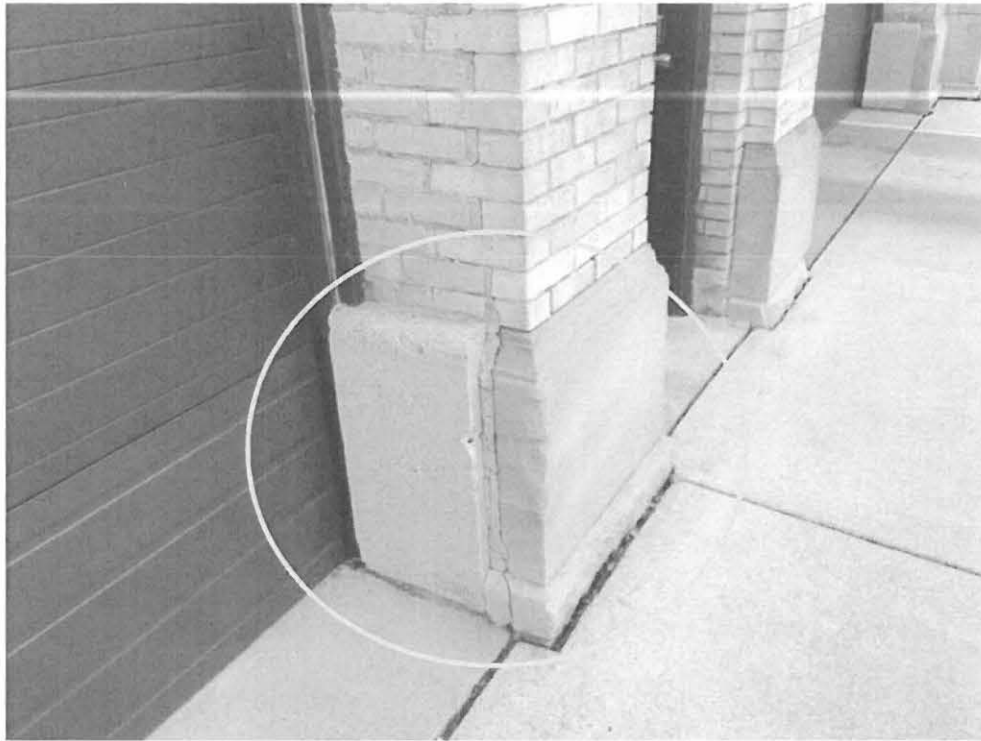
Figure 33: Stone deterioration.
