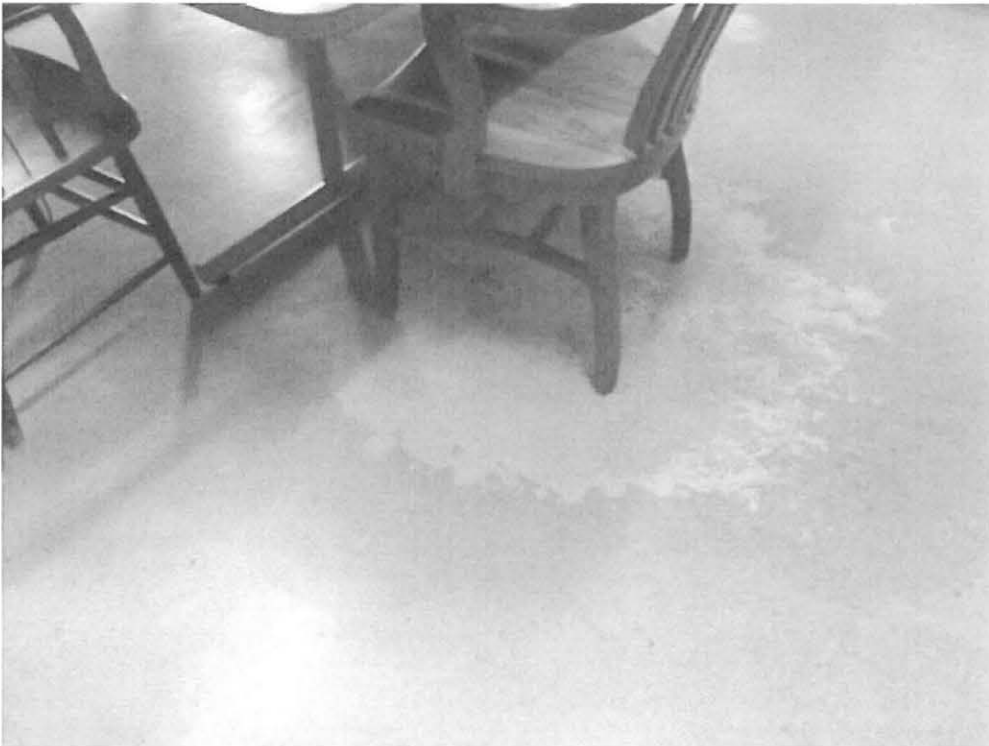
Figure 48: First floor concrete flooring.
