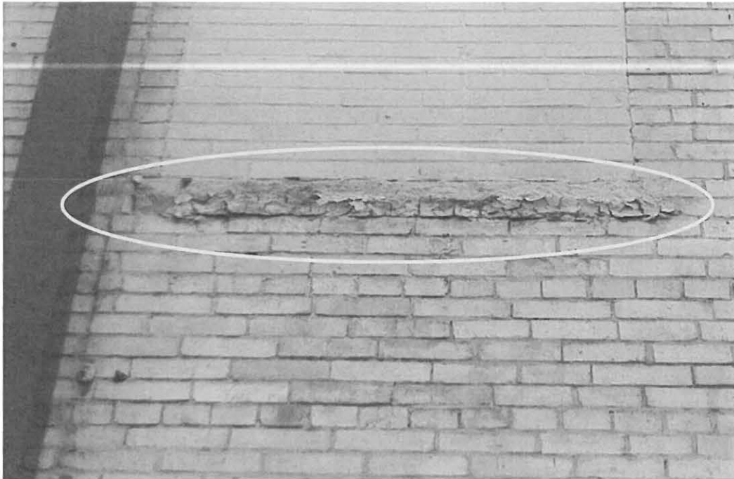
Figure 35: Deteriorated sill.
