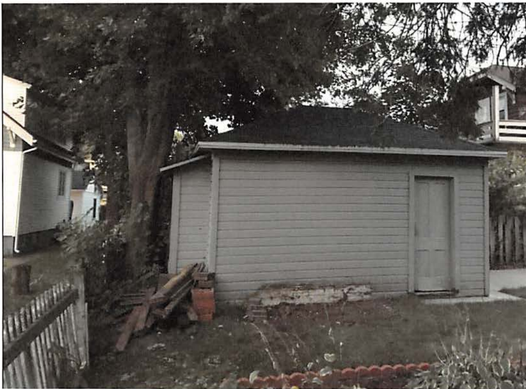
Figure 11- View of the current garage from the west looking east. The fence on the bottom left represents the property edge, however it has been pushed outward by the large tree behind the garage.
