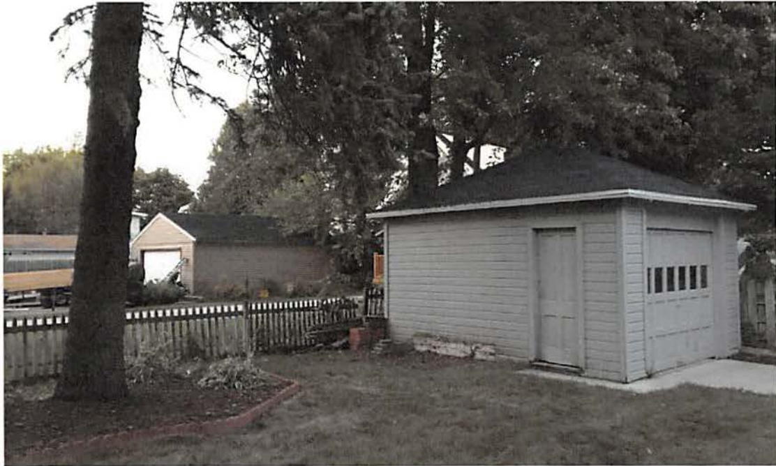
Figure 10 - View of the current garage and yard for garage expansion area from the southwest looking northeast
