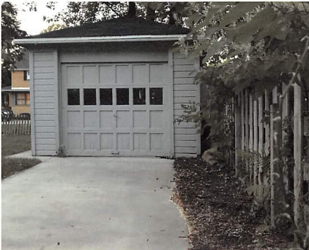
Figure 9 - View of current garage and proximity to the property line
