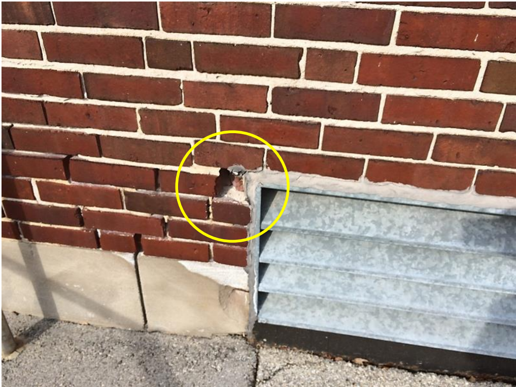
Figure 40: Cracked brick
