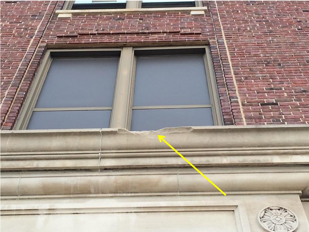
Figure 44: Spalled Stone
