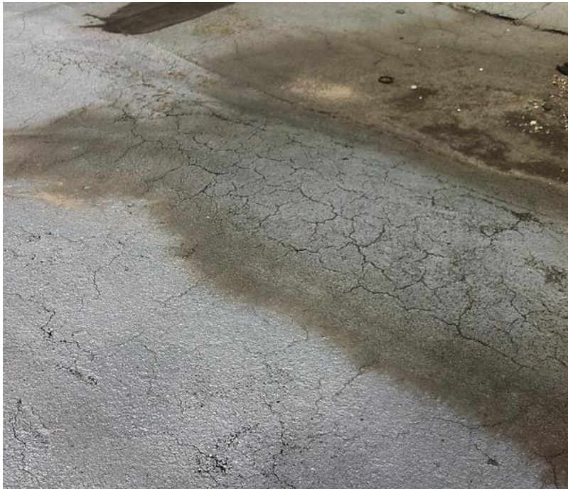
Figure 13: Membrane cracking.
