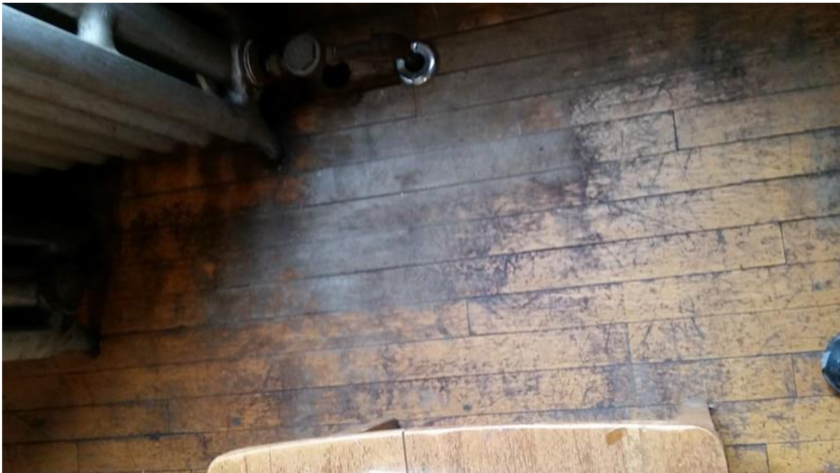
Figure 74: Fourth floor wood flooring
