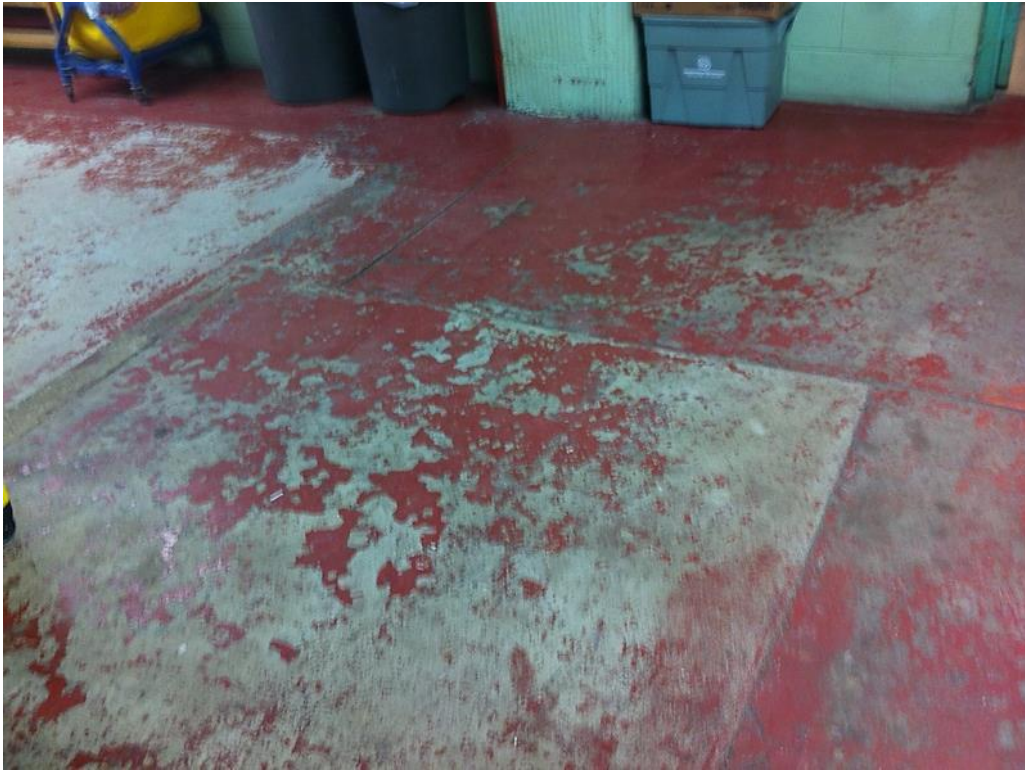
Figure 55: Basement concrete floor in boiler room
