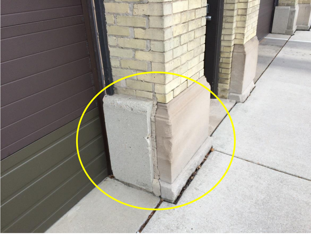
Figure 33: Stone deterioration.
