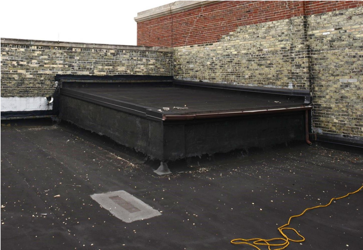
Figure 24: Roof area C
