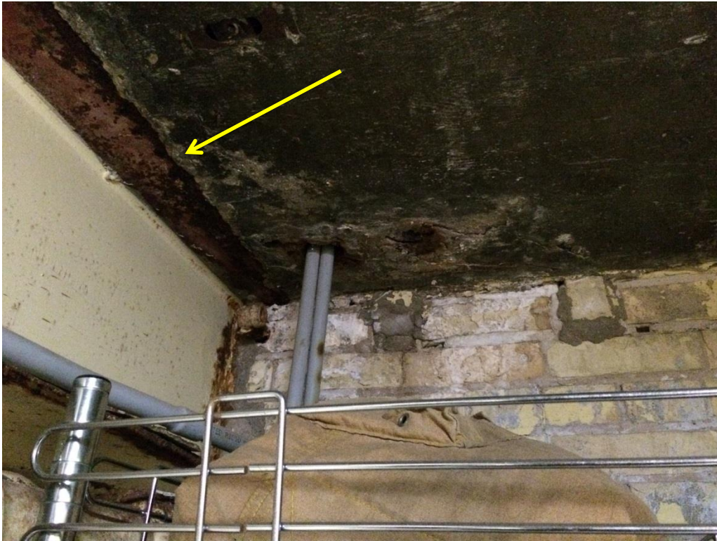
Figure 39: Steel Corrosion.
