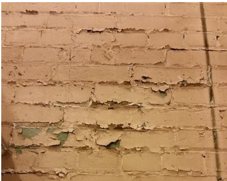
Figure 34: Paint deterioration.
