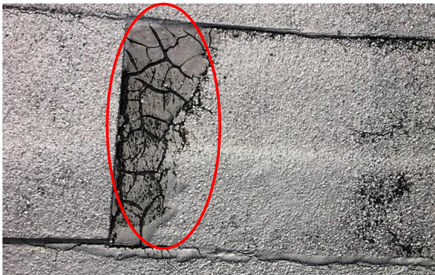
Figure 10: Alligator cracking.
