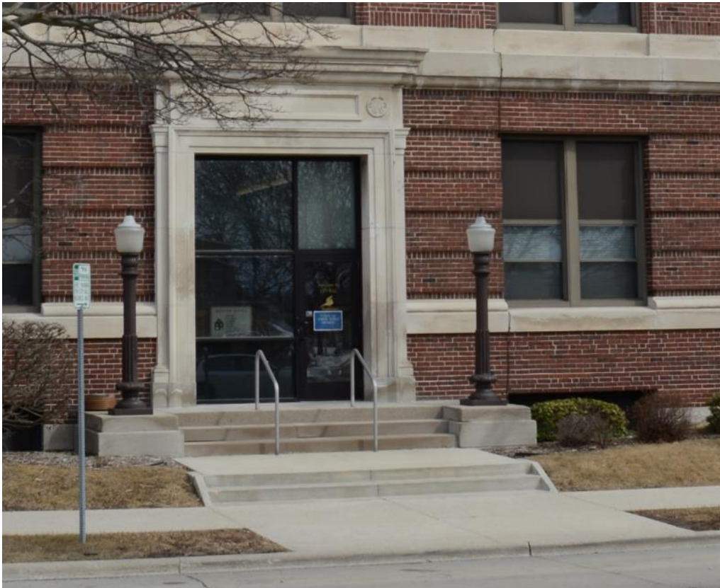
Figure 9: Typical entrance system, west facade
