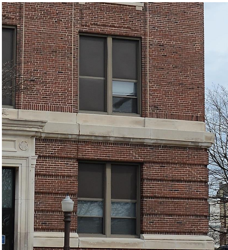
Figure 36: Typical brick coursing
