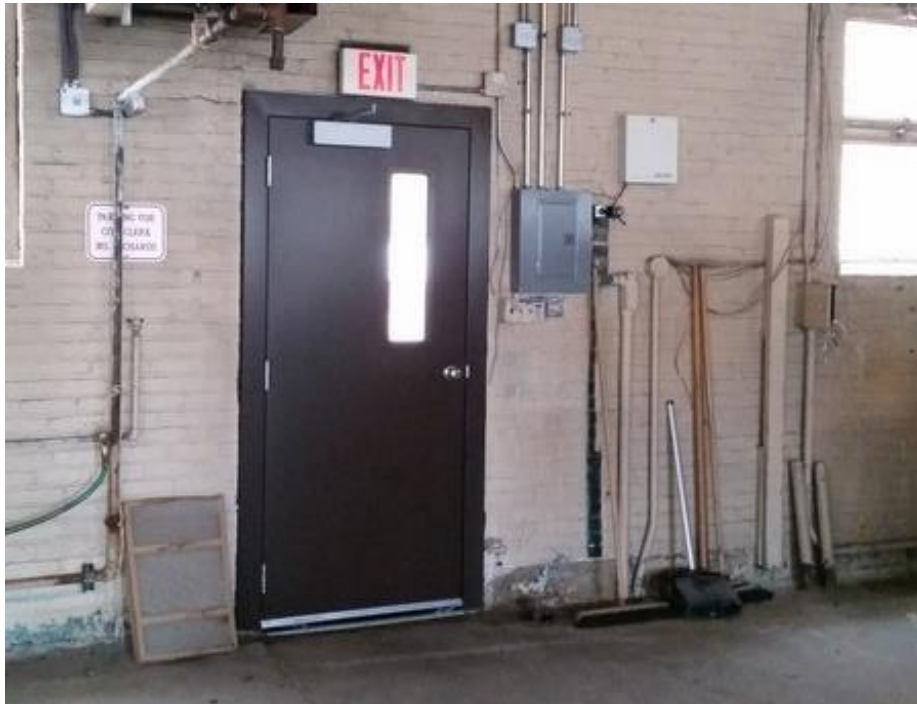
Figure 21: Interior view of south facade access door.
