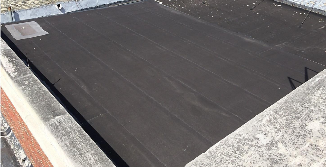
Figure 23: Roof area B
