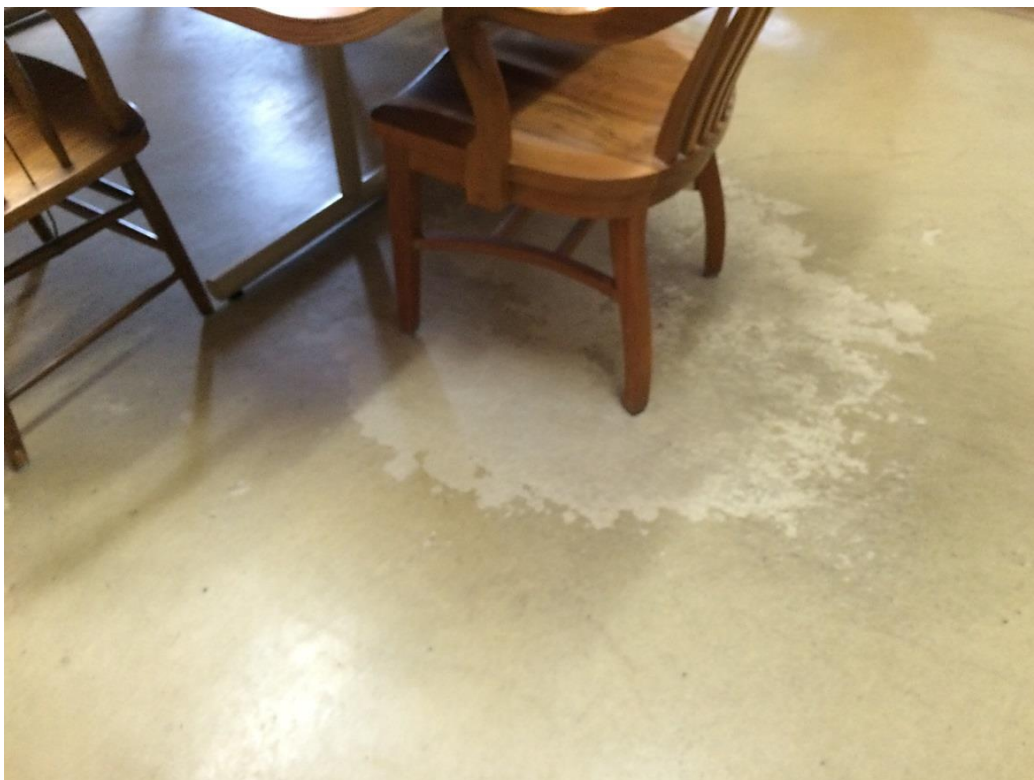
Figure 48: First floor concrete flooring.
