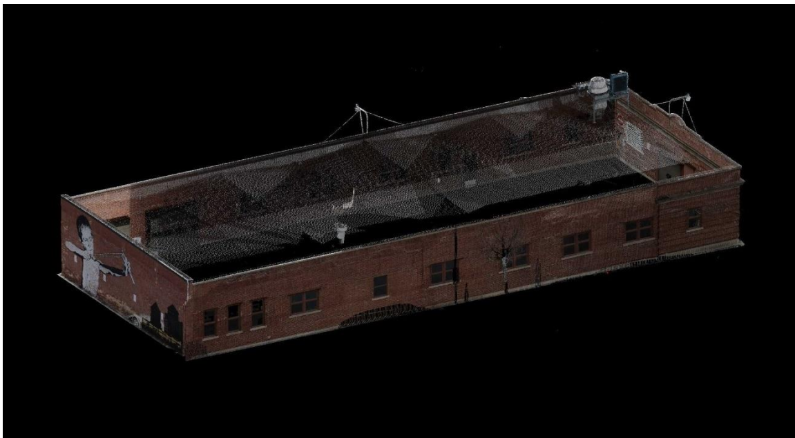
Figure 2: Sheboygan City Hall North Parking Garage colorized 3D laser scan image.
