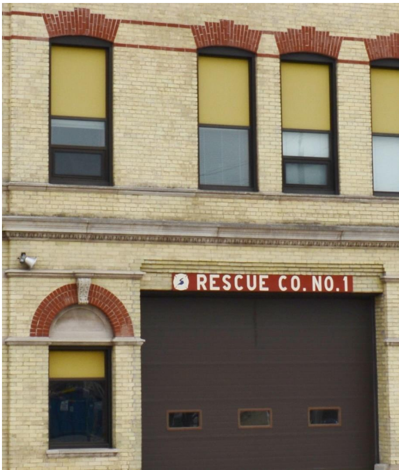
Figure 20: Typical window systems.
