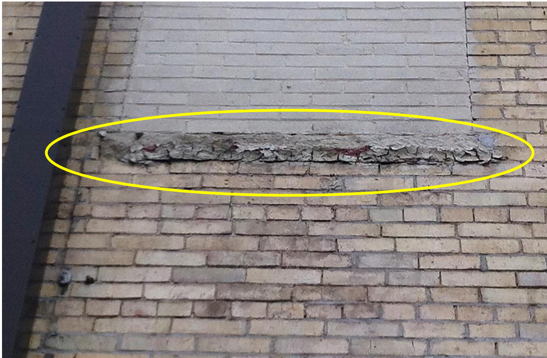
Figure 35: Deteriorated sill.
