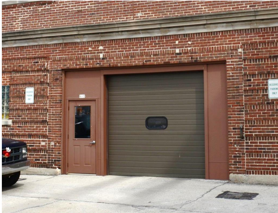
Figure 19: West facade doors.
