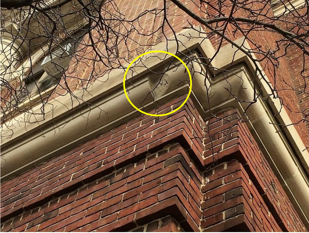
Figure 45: Spalled stone
