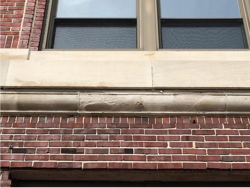
Figure 43: Stone erosion.
