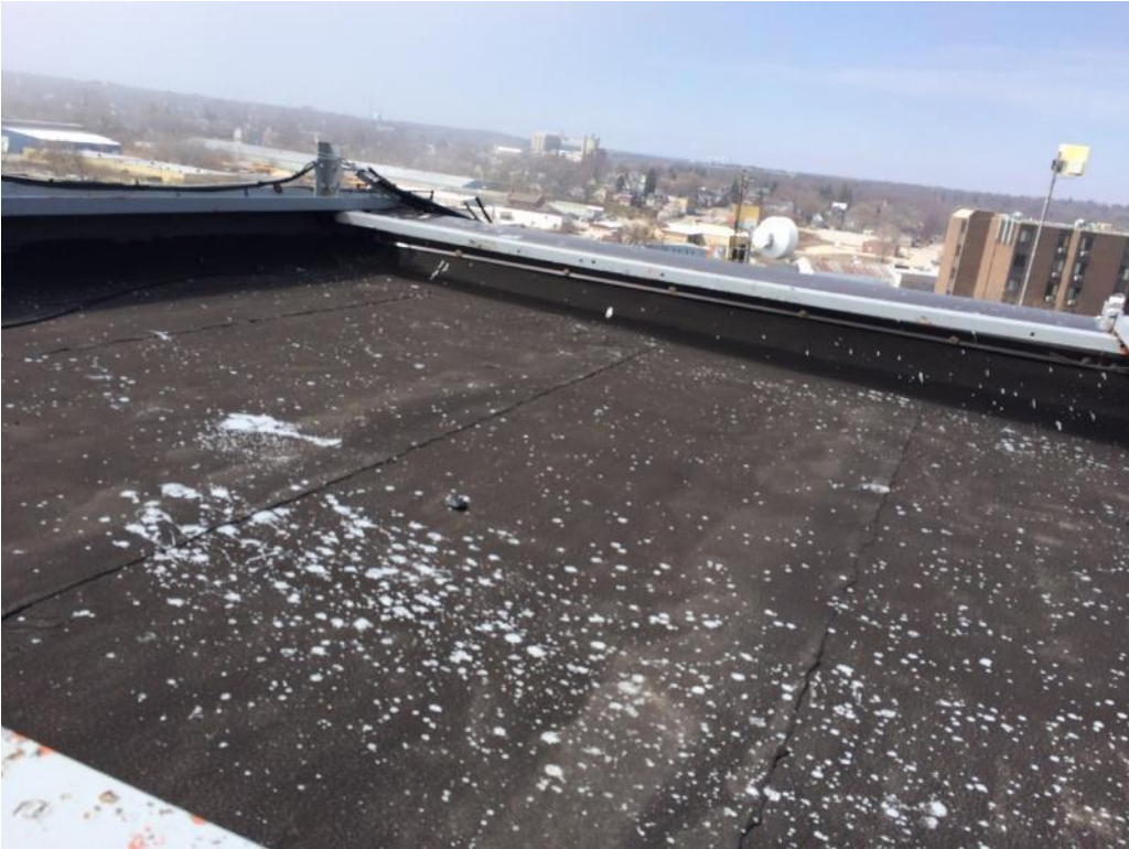
Figure 22: Roof area A
