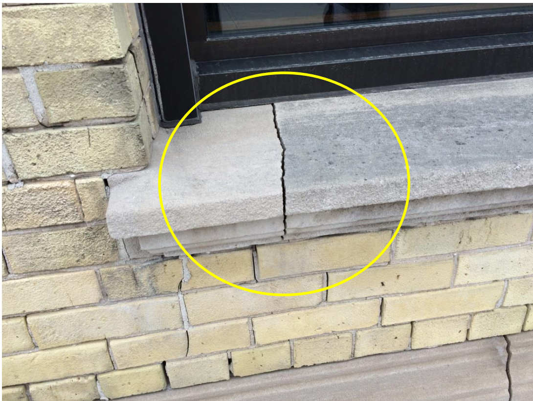
Figure 36: Cracked sill.
