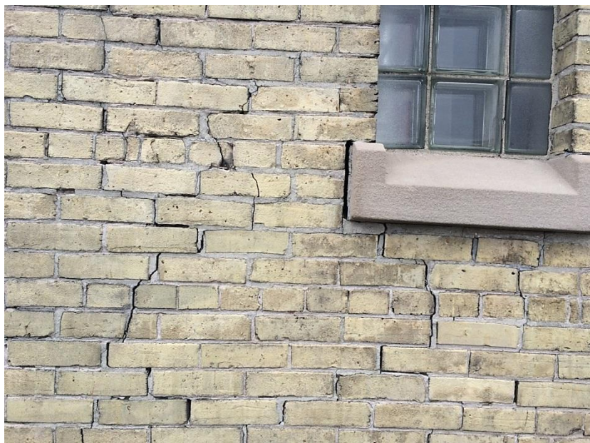
Figure 24: Brick/mortar cracking.
