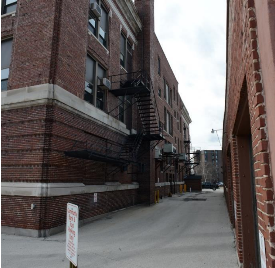
Figure 11: Alley, north elevation
