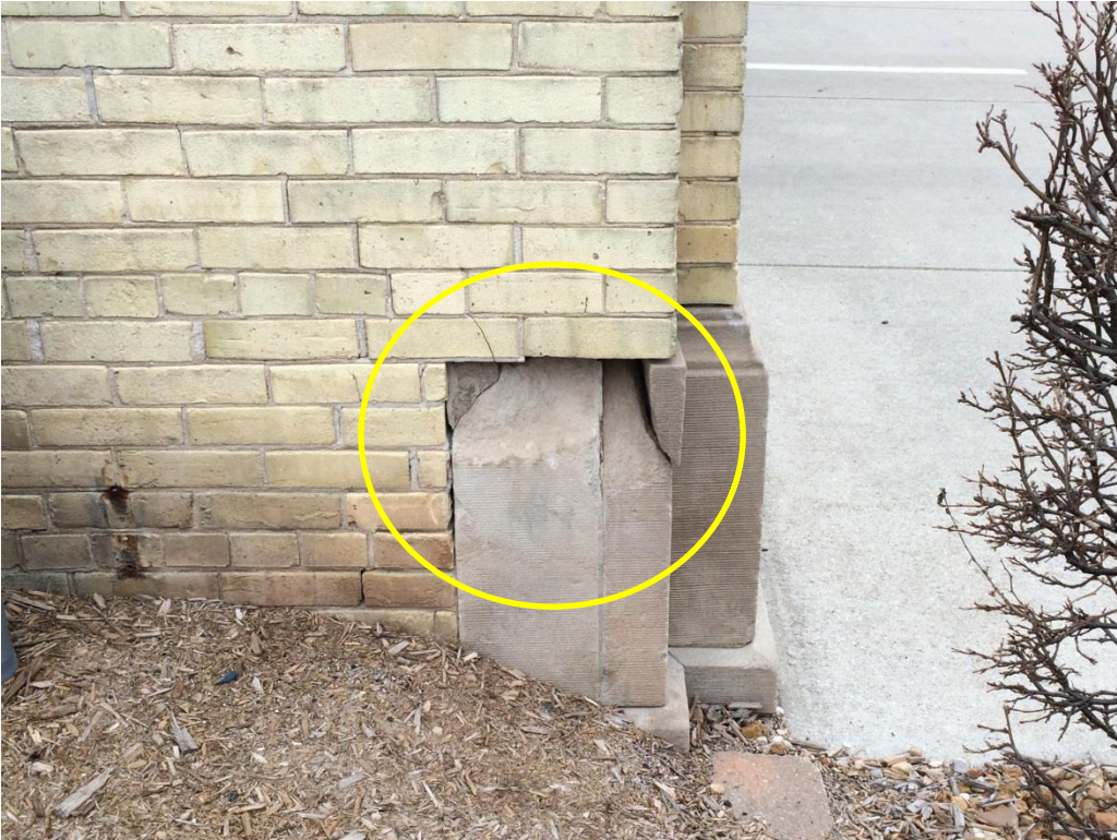
Figure 34: Stone spalling.
