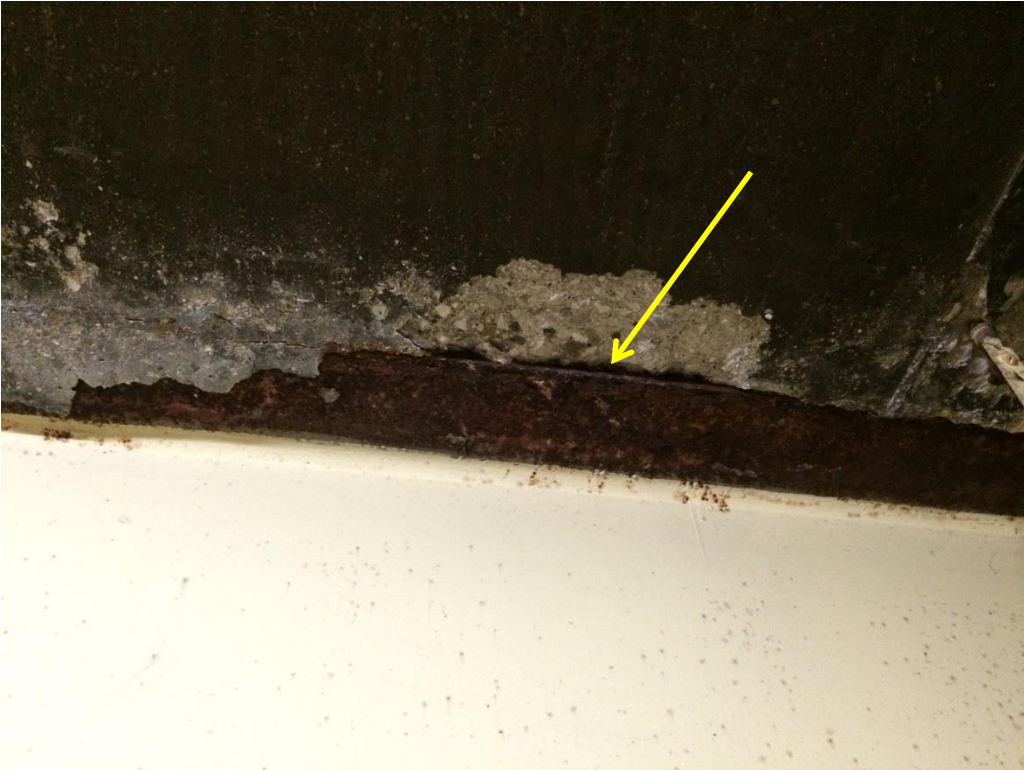
Figure 38: Steel corrosion.
