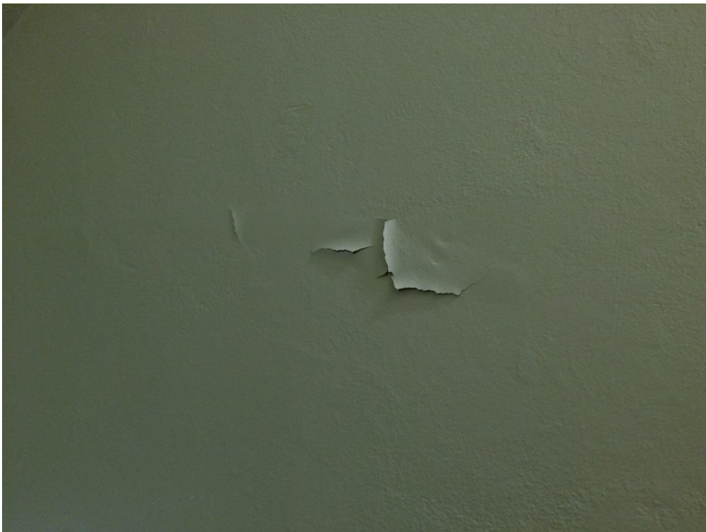
Figure 44: Paint failure.
