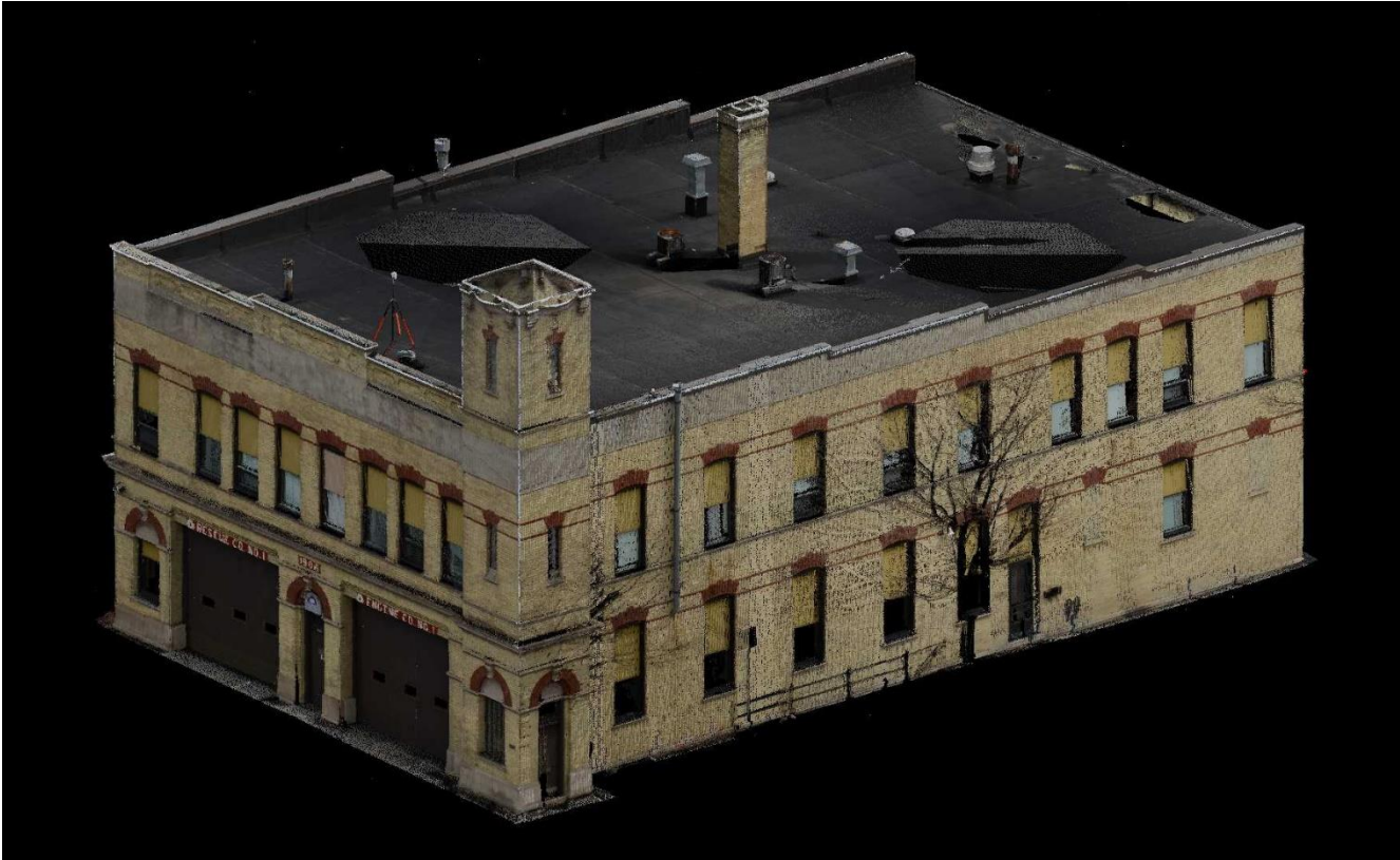
Figure 3: Sheboygan Fire Station No. 1 colorized 3D laser scan image.
