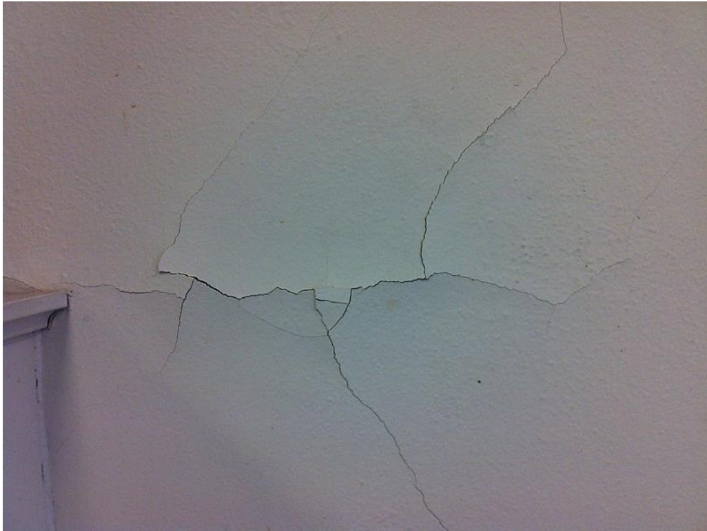
Figure 65: Paint cracking
