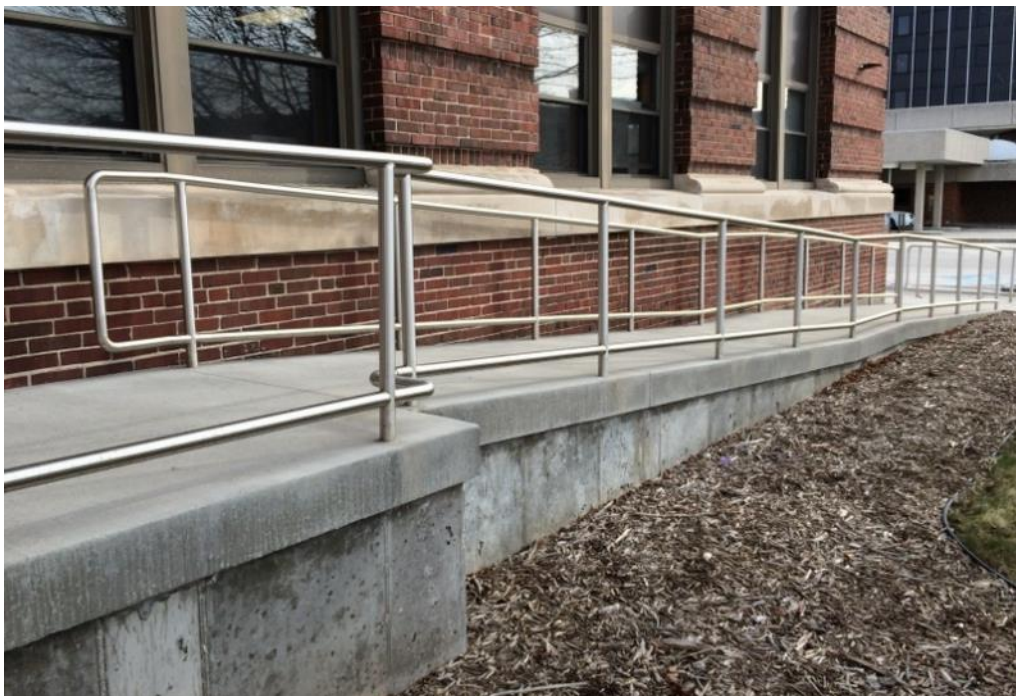
Figure 10: Wheelchair ramp entrance, south facade
