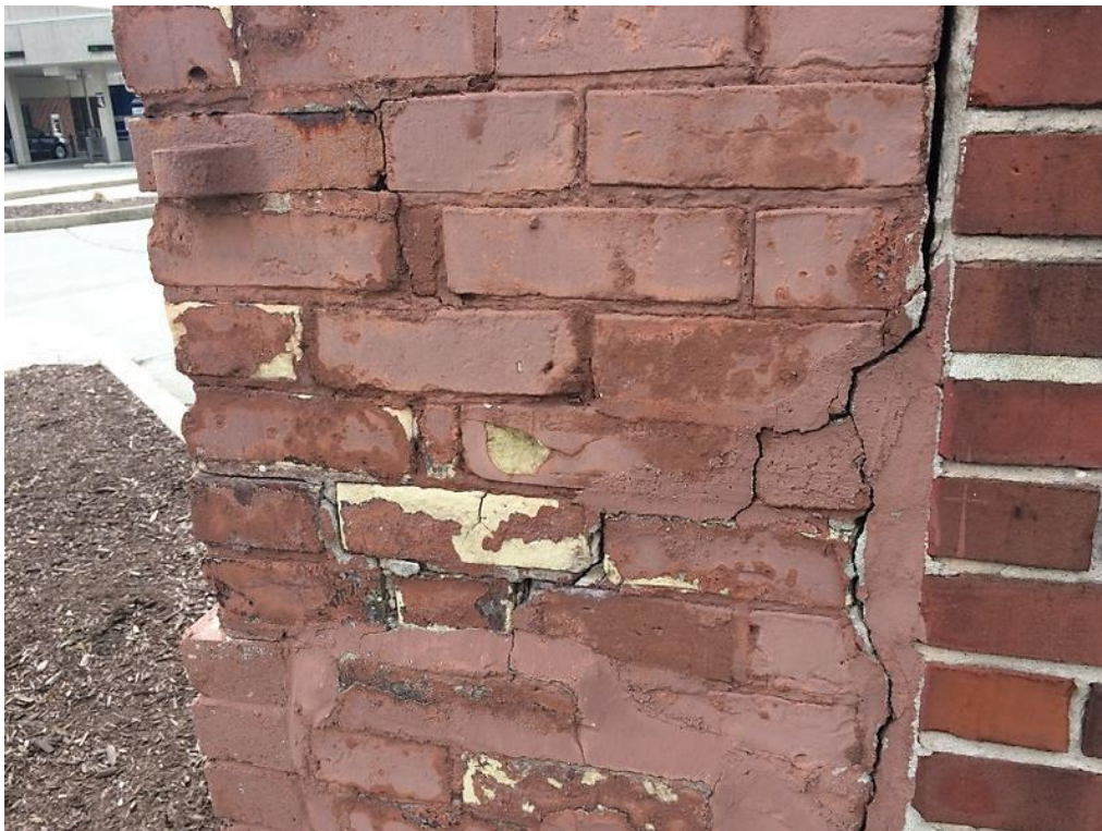
Figure 24: Deteriorated brick.
