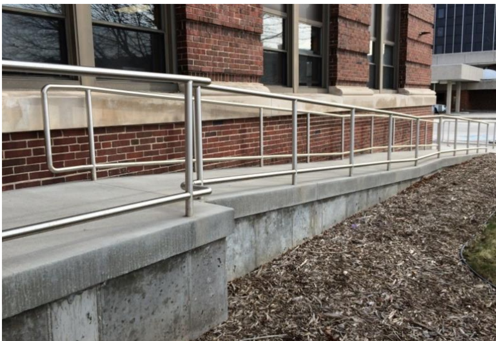
Figure 10: Wheelchair ramp entrance, south facade
