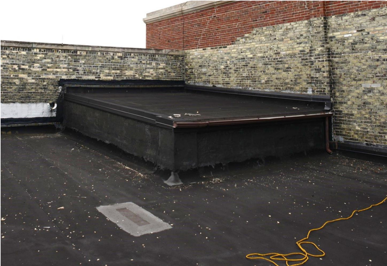
Figure 24: Roof area C
