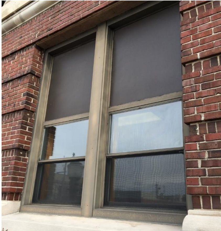
Figure 29: Typical window system
