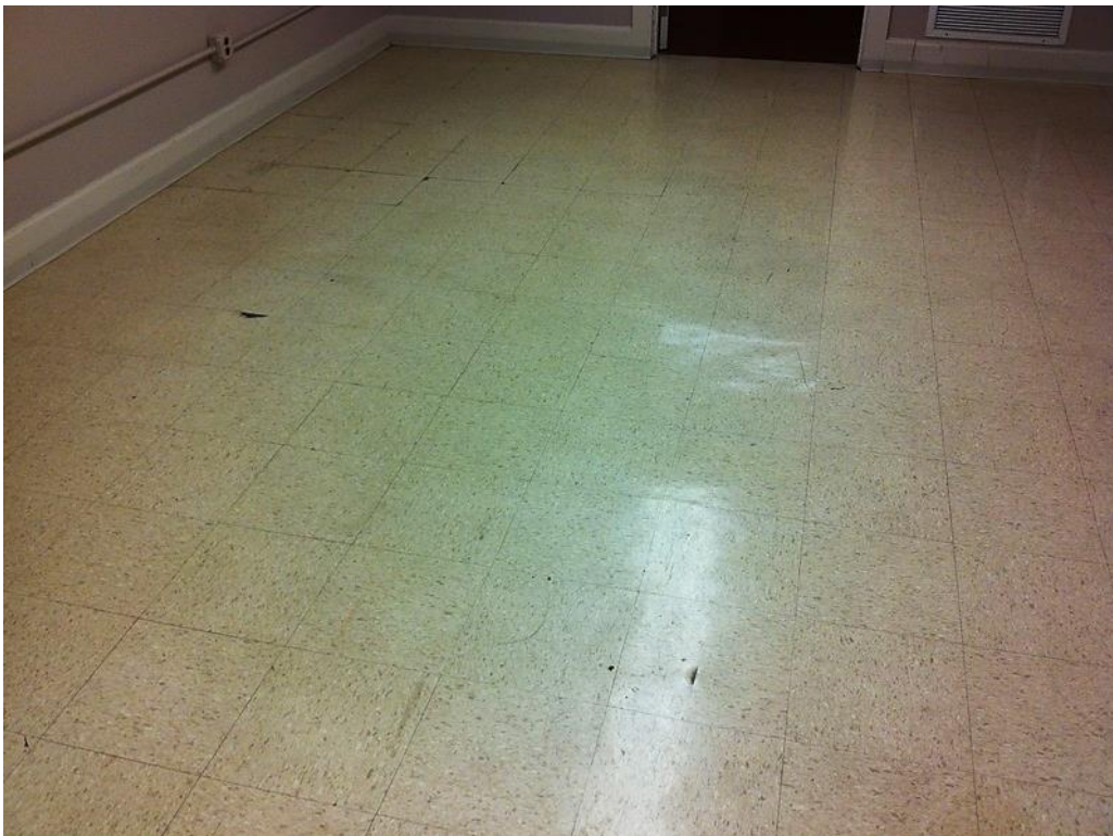
Figure 52: Basement common area tile
