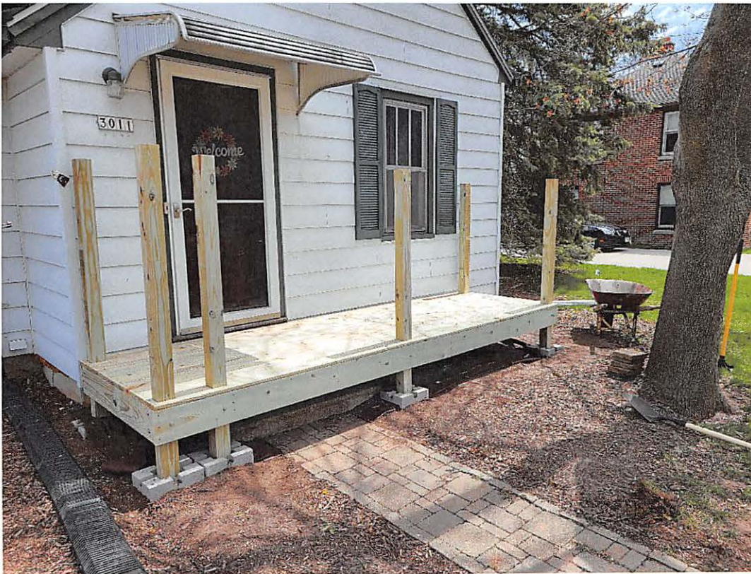
An additional 2 legs were added to support the left side railing bringing the total to 7 legs. 14ft deck boards were added to create a walking surface that lines up perfectly with the front door.
