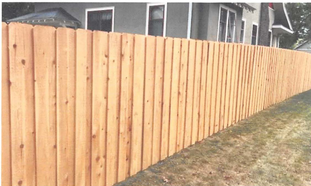
Figure 2: Example unstained board on board design. Image provided by Whirl Wind Post Holes & Fencing.
