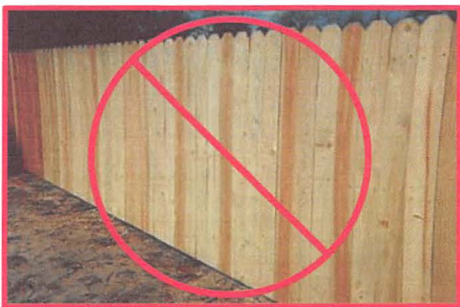
Figure 3: Example of flat dog-ear. Not the design intent. Image provided by A Murphy Fence Co.
