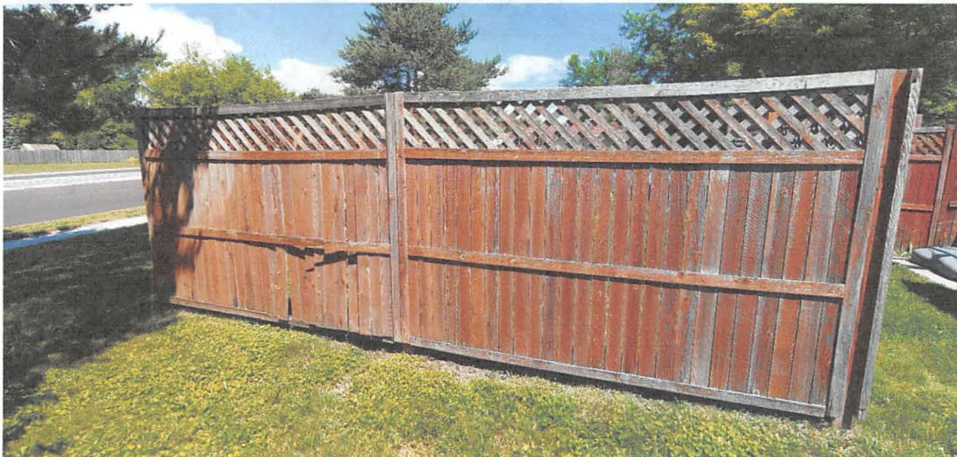
Figure 5: Greying and damage.
