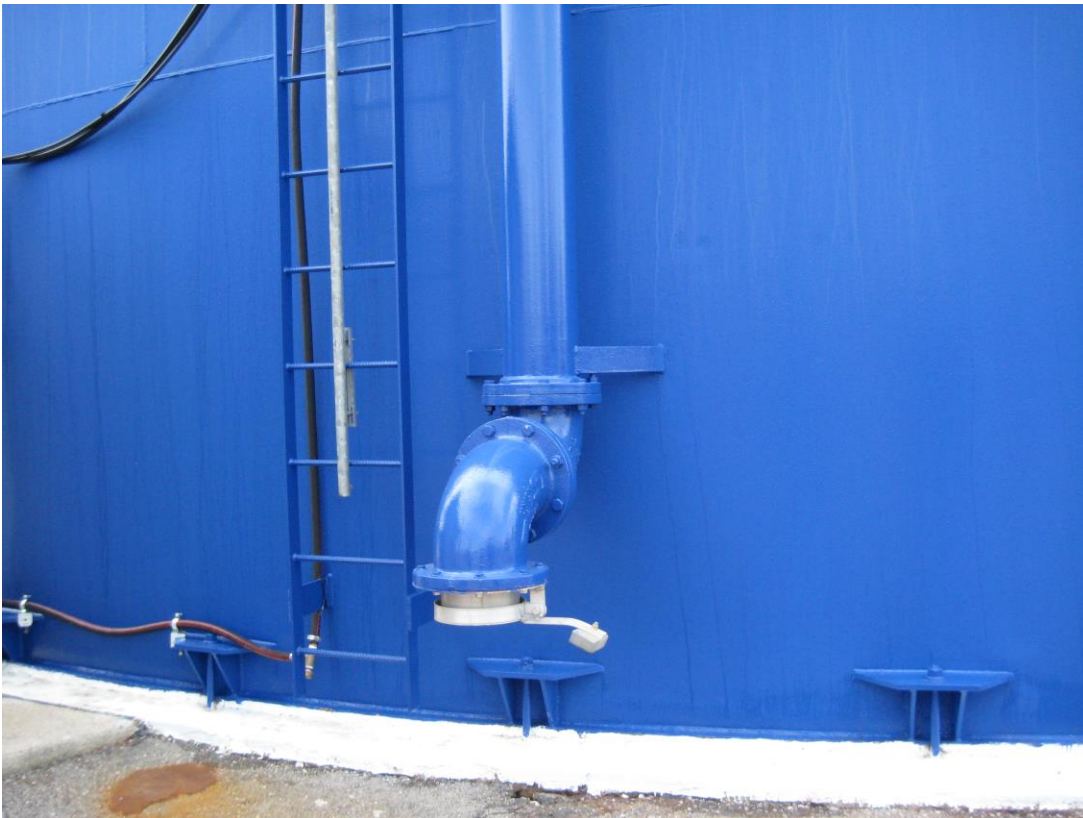
Georgia Avenue Standpipe
