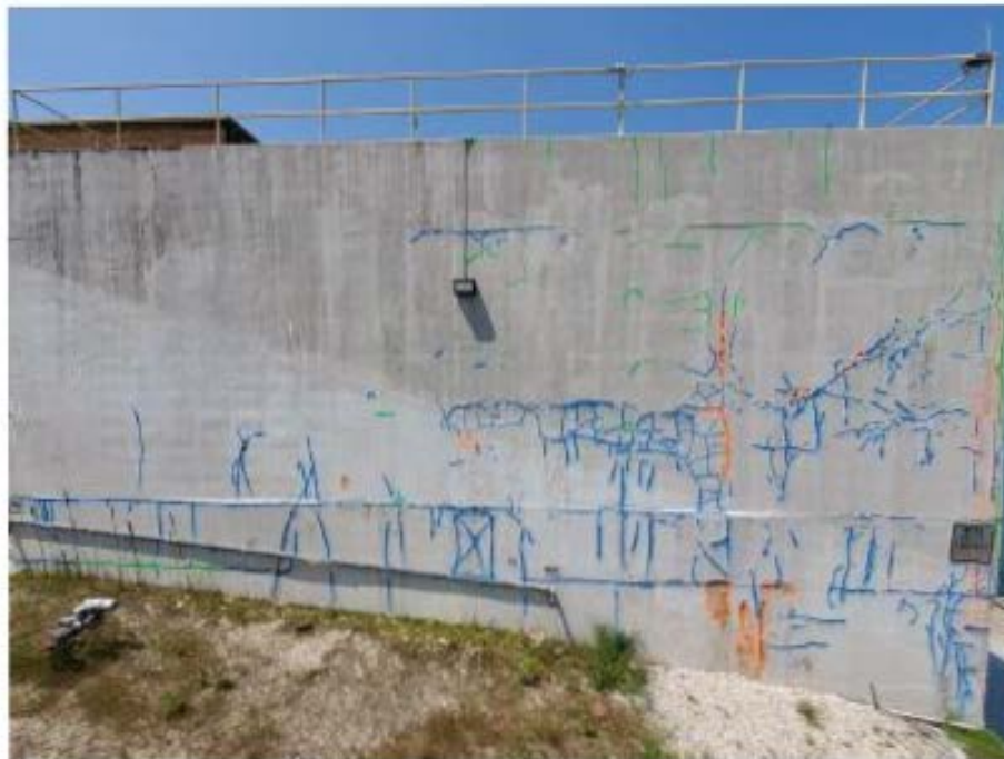
Photograph 40: 2020 Exterior inspection, south wall shown.
