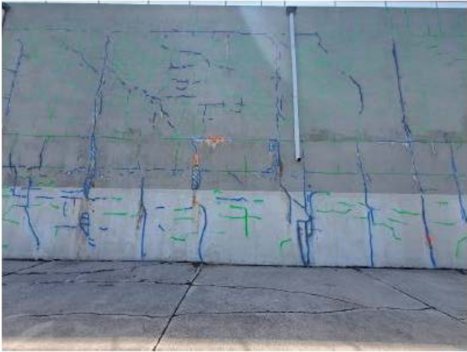
Photograph 37: 2020 Exterior inspection, scupper 4 and 5 shown.
