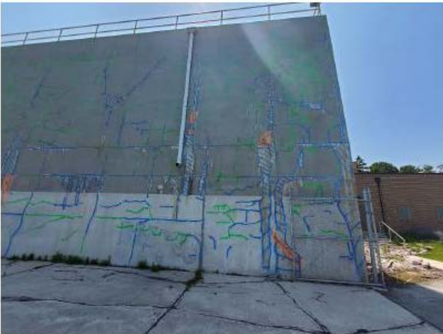
Photograph 32: 2020 Exterior inspection, north end to half panel past scupper 1.
