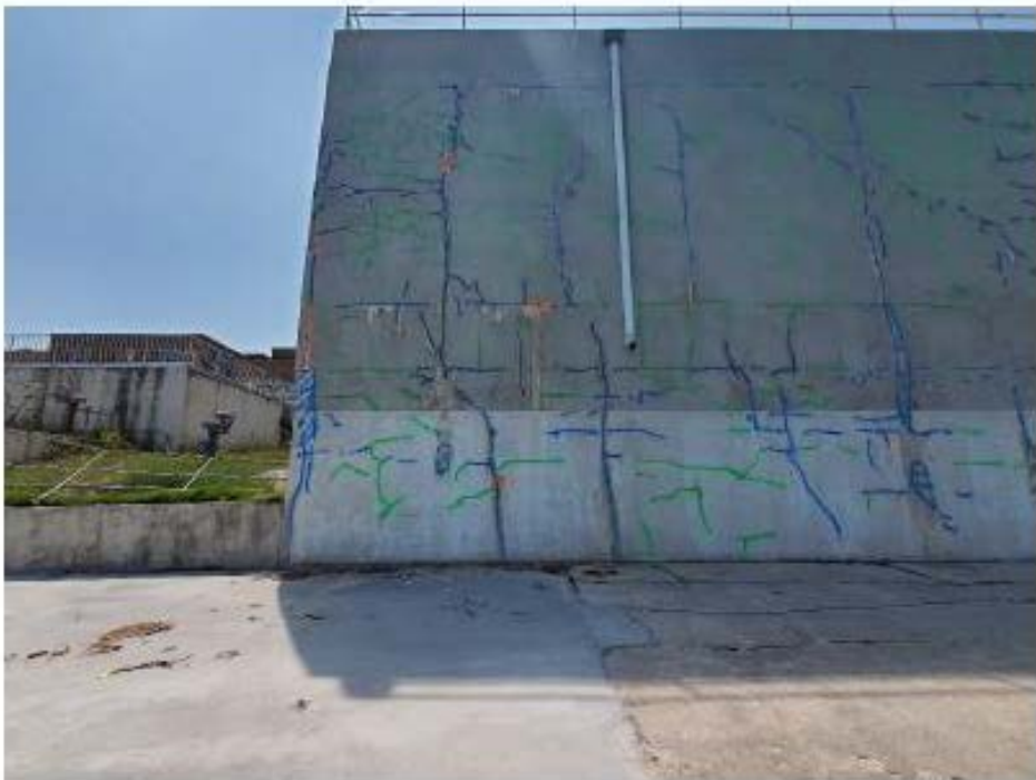
Photograph 38: 2020 Exterior inspection, south end to scupper 5 shown.
