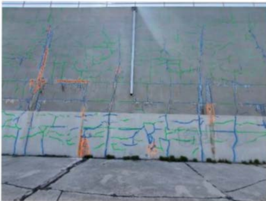
Photograph 34: 2020 Exterior inspection, half panel past scupper 2.
