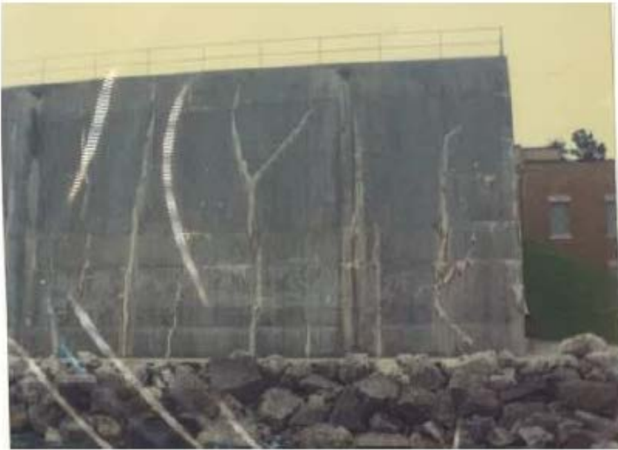
Photograph 31: 1993 Pre-repair photo, north end to scupper 2. .
