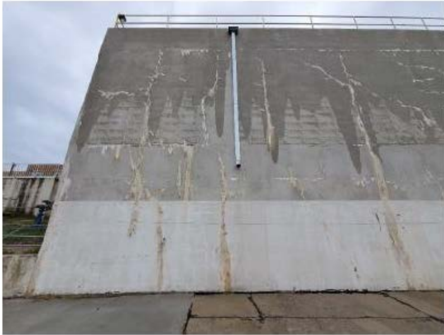
Photograph 11: Typical condition of exterior east wall. South end shown.
