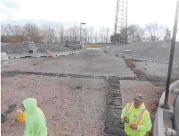
New Water Treatment Roof – Overview Photo
