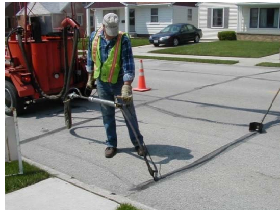
Street Excavation Patch
