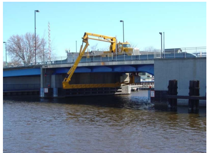
8 th Street Bridge being inspected
