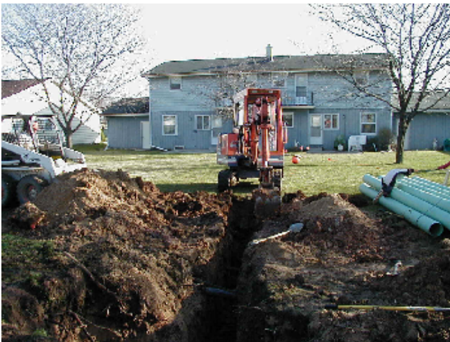
Mini-Storm Sewer Installation - Backyard
