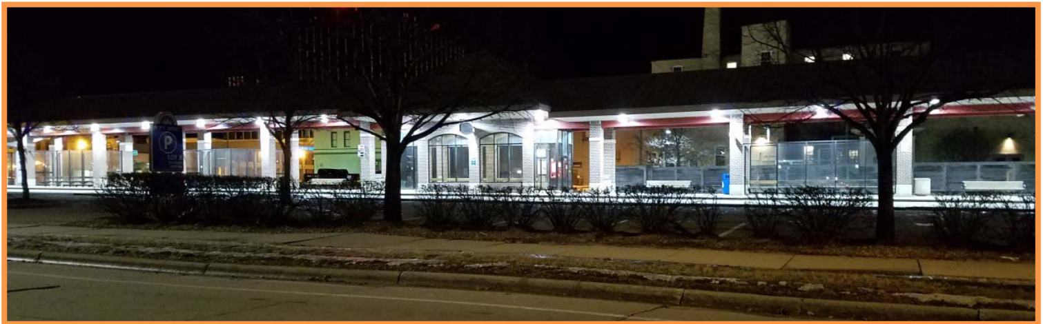
LED Upgrade at the Sheboygan Transit Transfer Station
