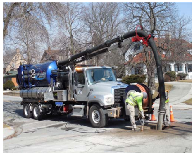
Sewer TV Crew
