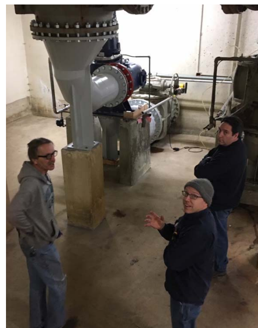
Installation of new Raw Influent Pump
