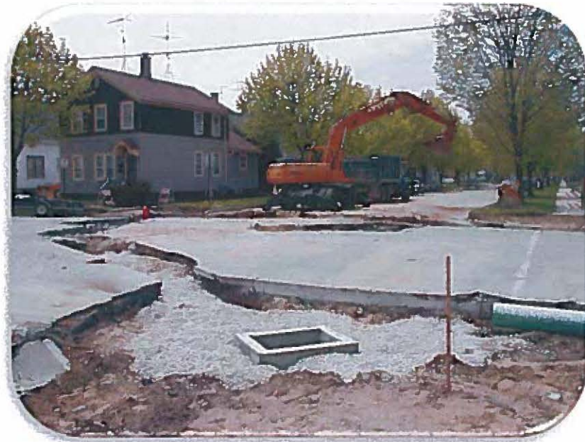
Storm Drain (Catch Basin) Installation
