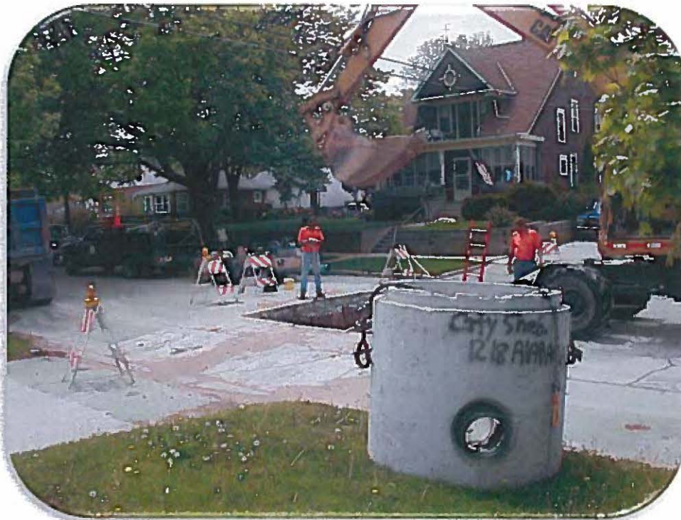
Precast Manhole with Rubber Boot
