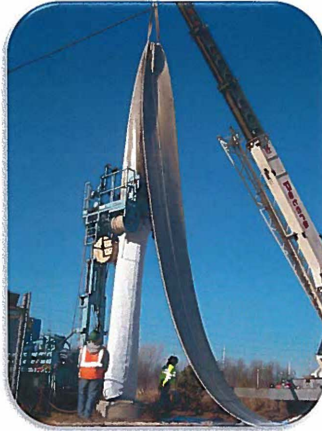
Liner Being Inserted Into Sewer Pipe
