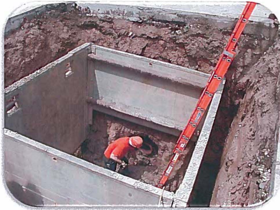
Preparing to Install a New Sanitary Manhole
