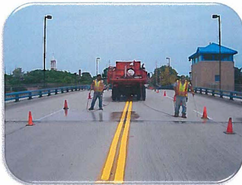
8th Street Bridge deck being seal coated (County Highway Shared Service)
