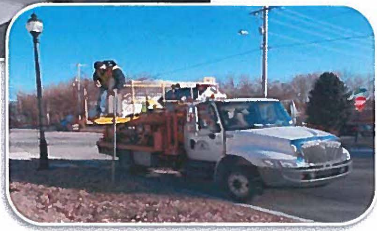
Installation of Signs
