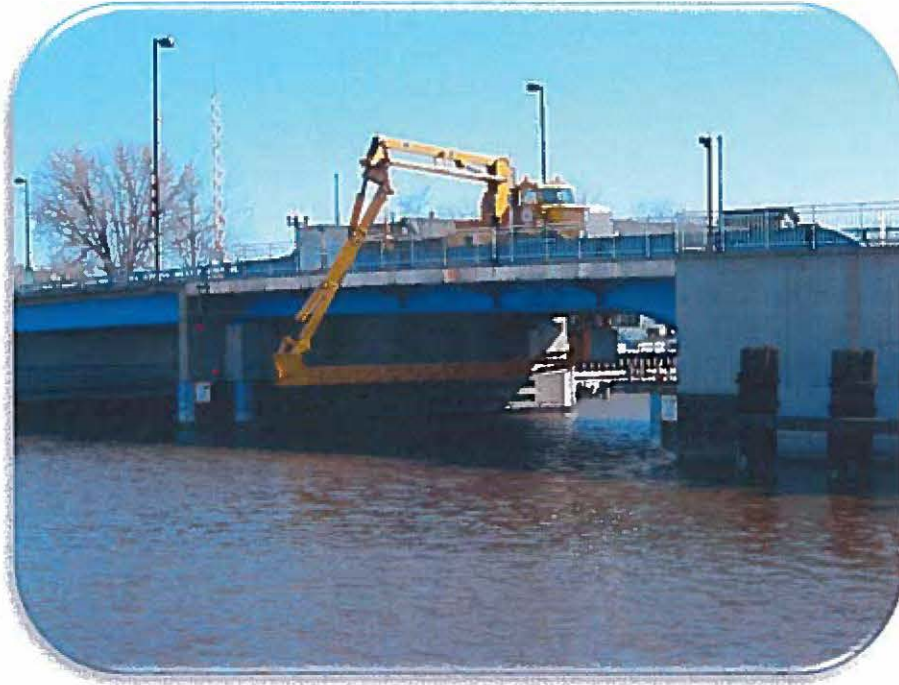
8th Street Bridge being inspected
