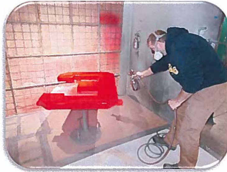
Fire Station #3 – Special Project
