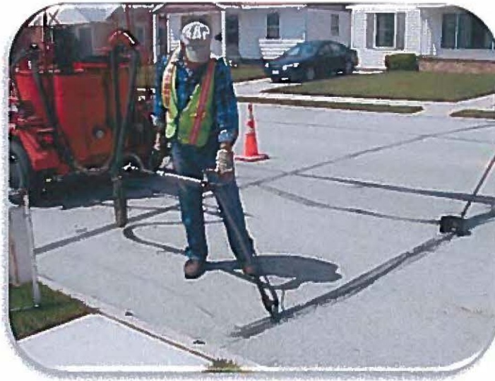
Crack Filling on Asphalt Overlay
