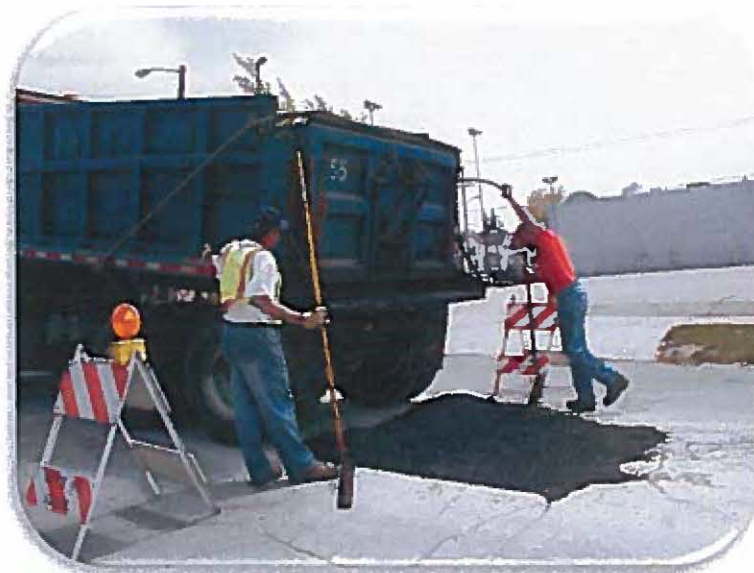
Street Excavation Patch
