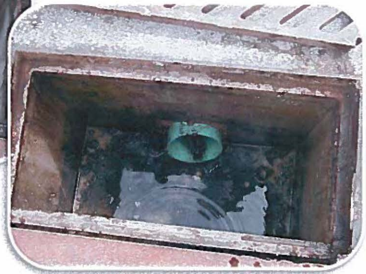
Catch Basin after Cleaning
