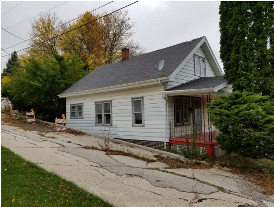
View of the subject from the alley way.
