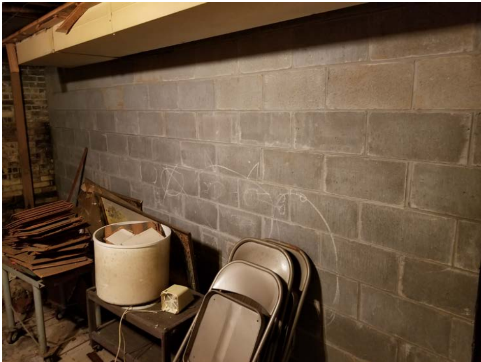
View of the subject repaired basement wall.
