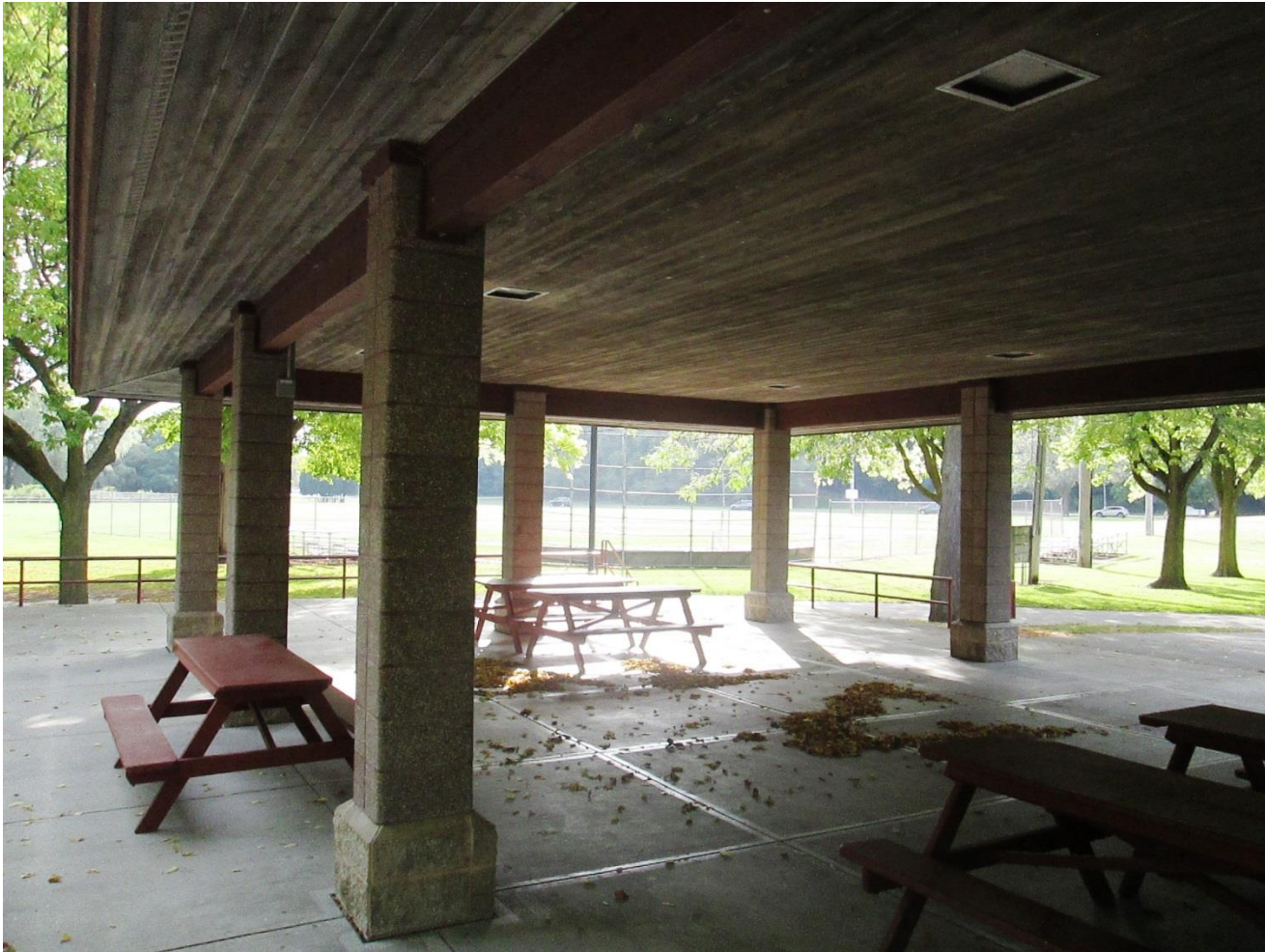
View of Main Shelter canopied area looking south/southwest
