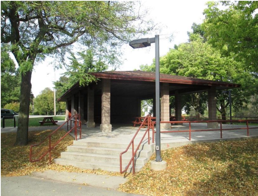
View of Main shelter looking North/Northeast from paved promenade
