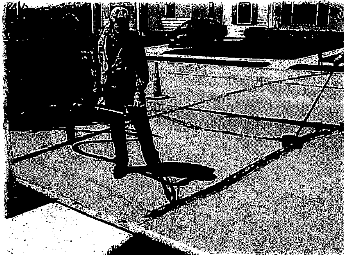
Crack Filling on Asphalt Overlay
