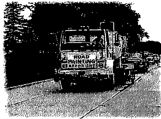
Street Centerline Painting (County Highway Shared Service)
