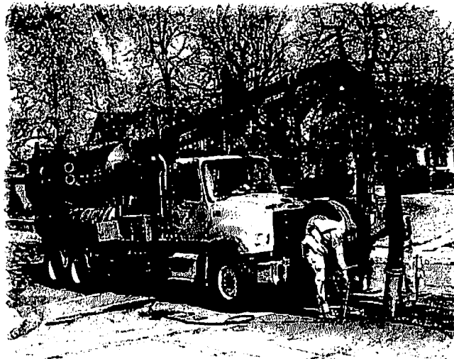
Sewer Vactor Truck
