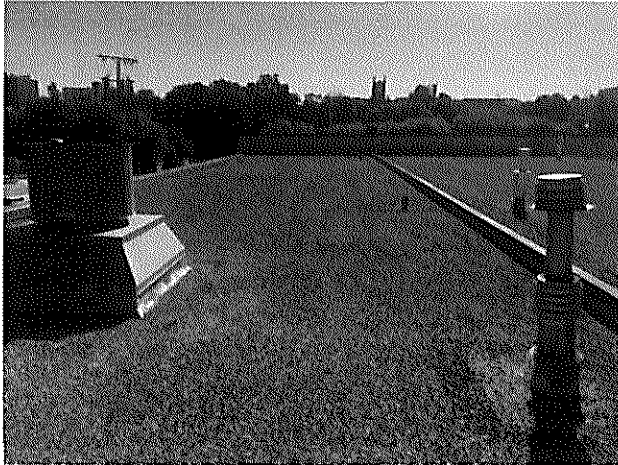
Transit Garage - Roof #4 – Overview 1
