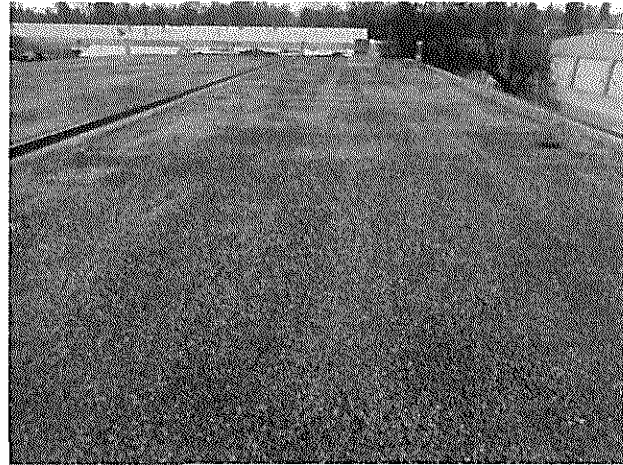
Transit Garage - Roof #4 – Overview 2
