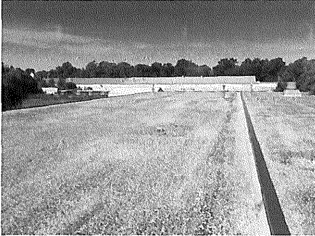
Transit Garage - Roof #5 – Overview Photo
