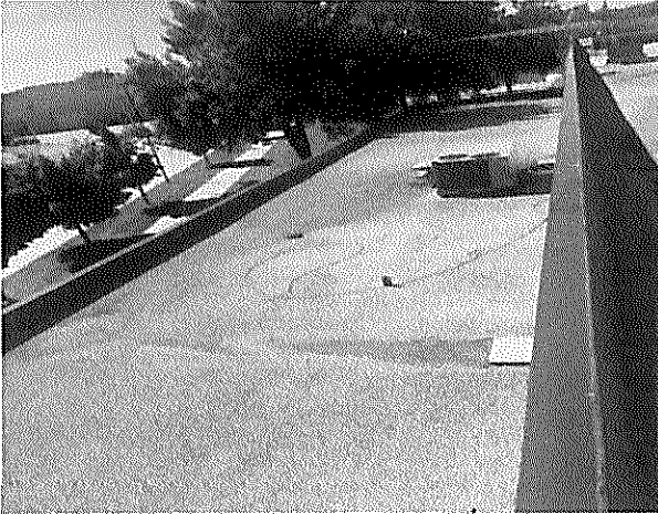
Transit Garage – Roof #1 - Overview
