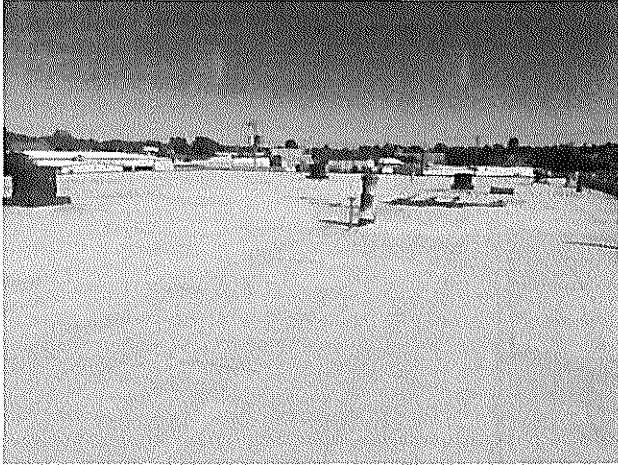
Transit Garage - Roof #2 – Overview Photo
